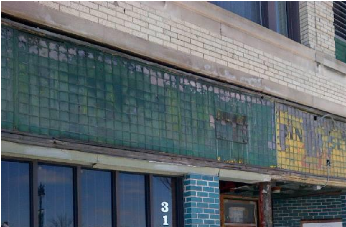
Prism glass above two storefronts at 3153 Woodward. This photo was taken in 2014, shortly as the removal of the non-historic awning, Staff believes that these transoms date from the building's original construction. Source, Joel Landy
