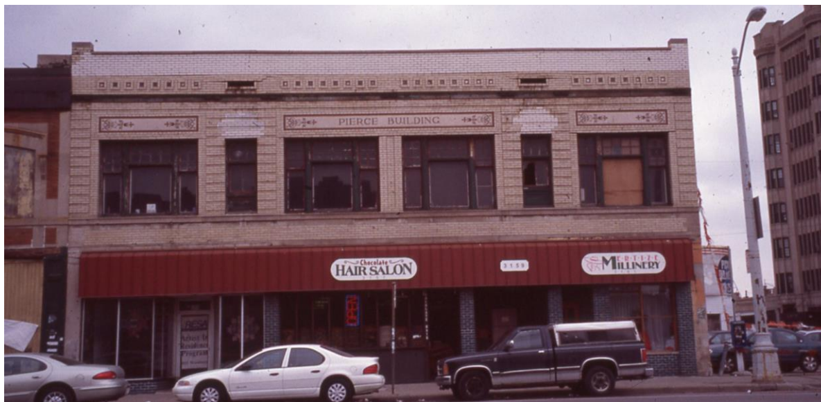
3153 Woodward, HDAB designation slide, appearance in 1984. Note that original wood windows are present at second story
