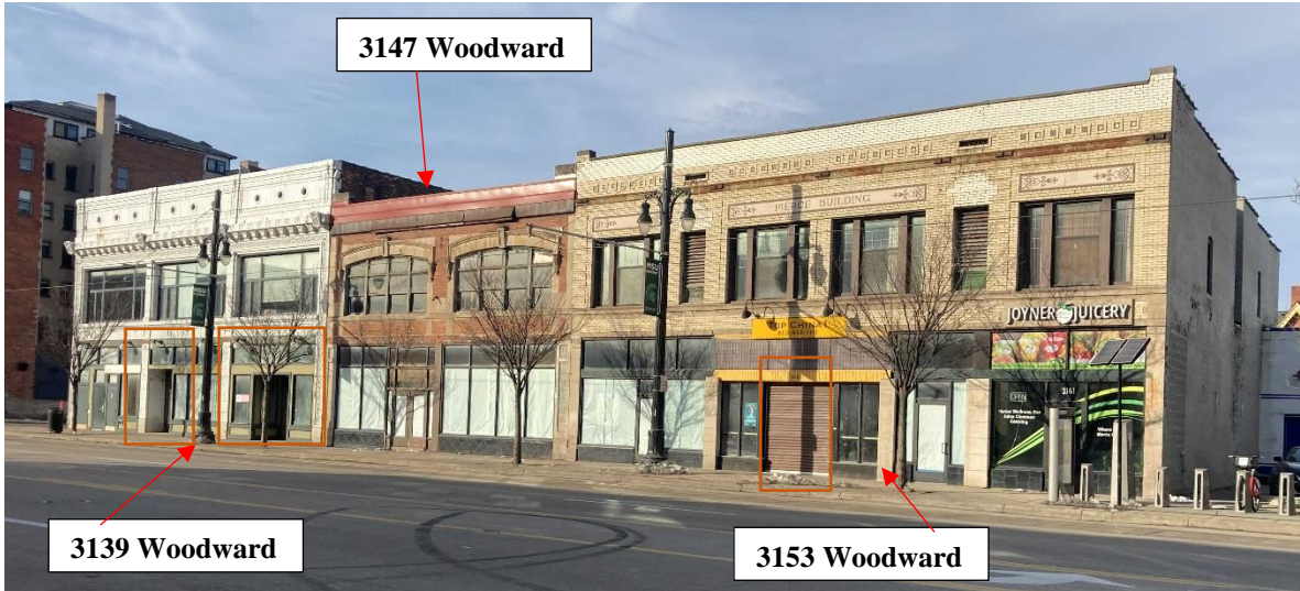
Current conditions, facing southwest showing 3139 Woodward (left), 3147 Woodward (center), and 3153 Woodward (right). Photo taken by HDC staff on 3/26/2024. Areas outlined in orange indicate areas where entry insets will be eliminated/project forward, flush with the sidewalk.
