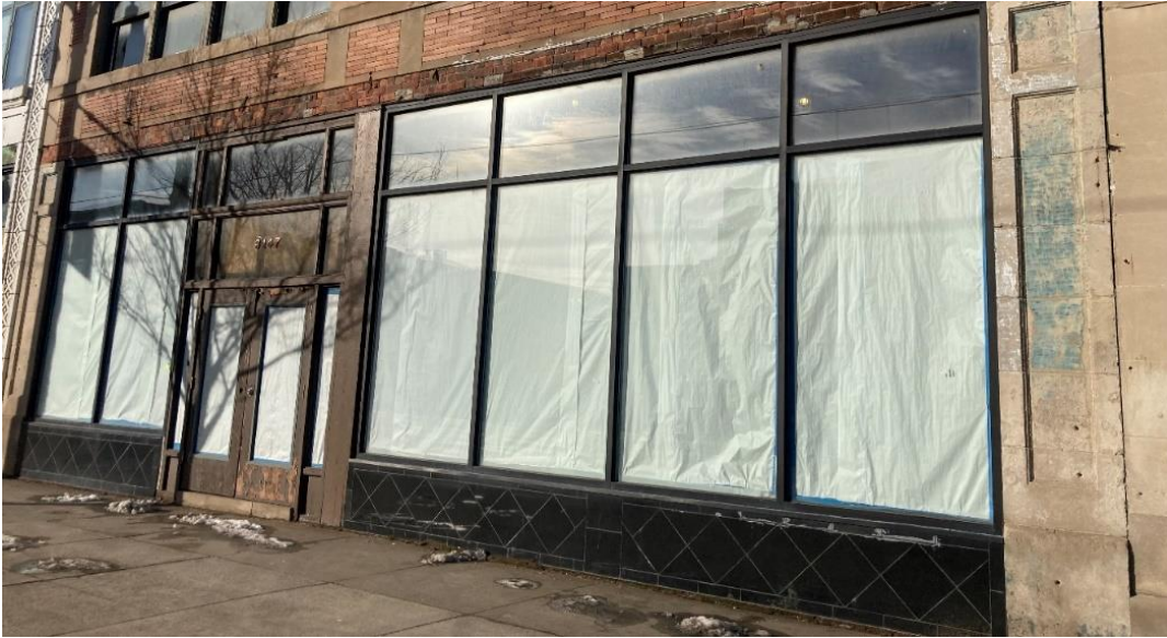
3147 Woodward, current appearance. Note that all portions of the storefront are new and that the above elevation drawing refers to “existing historic glass to remain and be restored.” Also, the configuration of the storefront does not match the approved. HDC staff photo taken on 3/26/2024, facing southwest
