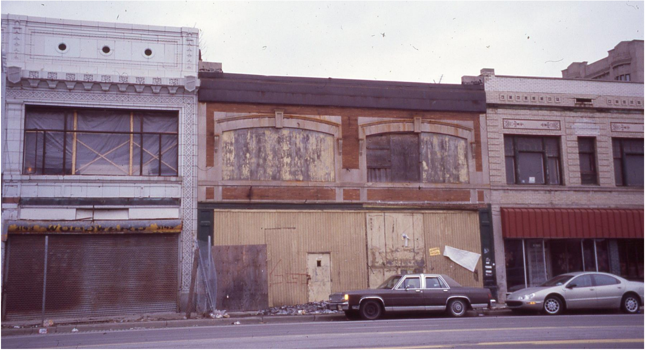
3147 Woodward (center), 3139 Woodward (left), and 3153 Woodward (right). HDAB designation slide, appearance in 1984. Note that new windows are in the process of being installed and storefront openings are covered.
