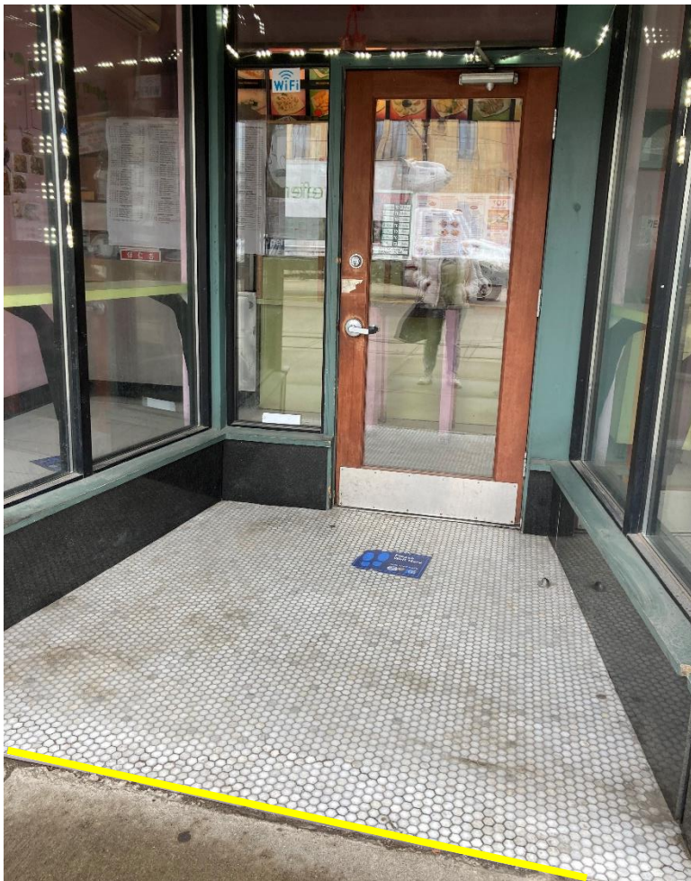
Single remaining inset entrance at 3153 Woodward. The inset and historic hex/penny tile floor will be removed as the new storefront will be located flush with the sidewalk. The yellow line indicates where the new storefront will be located. Note that none of the actual storefront material is historic age. Only the flooring and the inset placement of the door is historic. Staff photo taken on 4/4/2024
