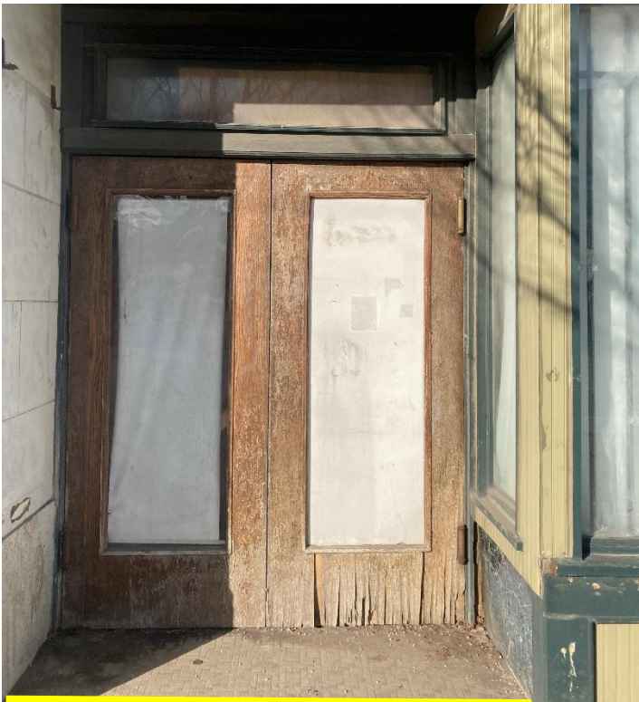
South remaining inset entrance at 3139 Woodward. Yellow line indicates where the new storefront will be located. The inset and historic tile floor will be removed as the new storefront will be located flush with the sidewalk. Note that none of the actual storefront material is historic age. Only the flooring and the inset placement of the door is historic. Staff photo taken on 3/26/2024
