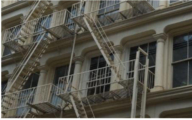
Example character-defining fire escape from the Landmarks Preservation Commission guidelines.
