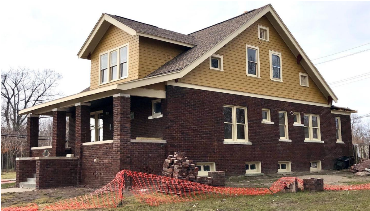
NE corner of house, view looking southwest from Garland.
