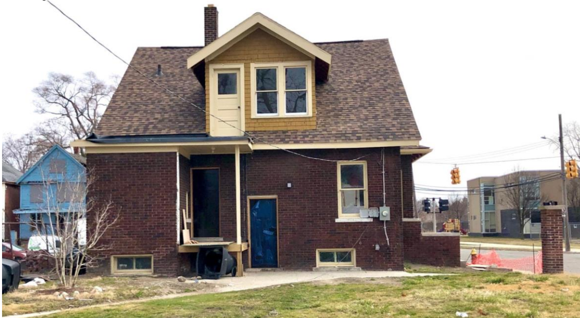
Rear (west) wall.
