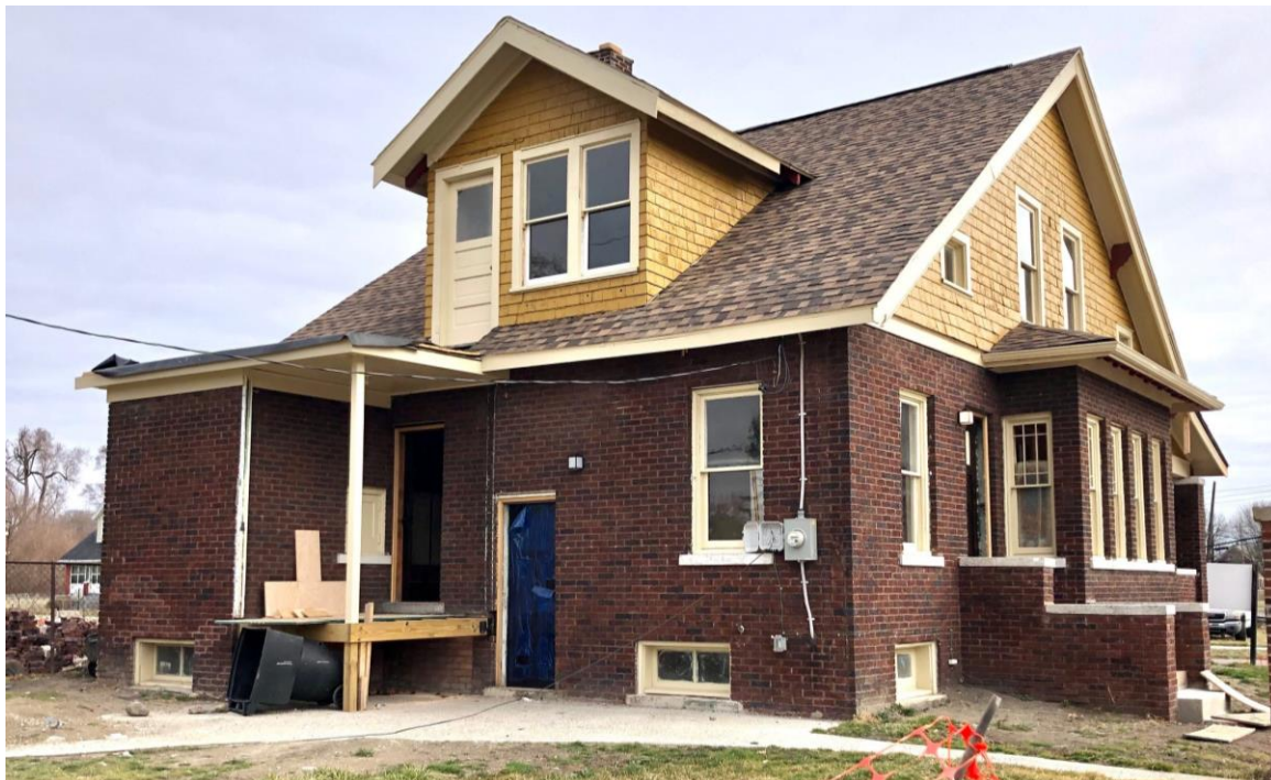
SW corner of house, from Charlevoix looking northeast.
