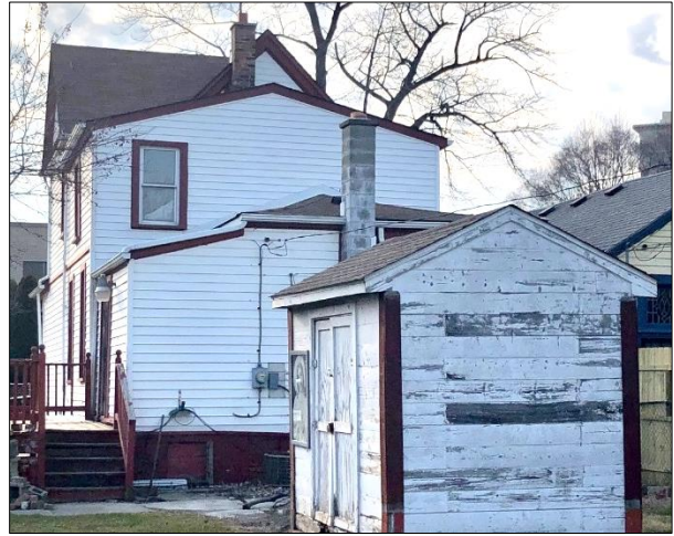
Above: Existing conditions at rear elevation.
