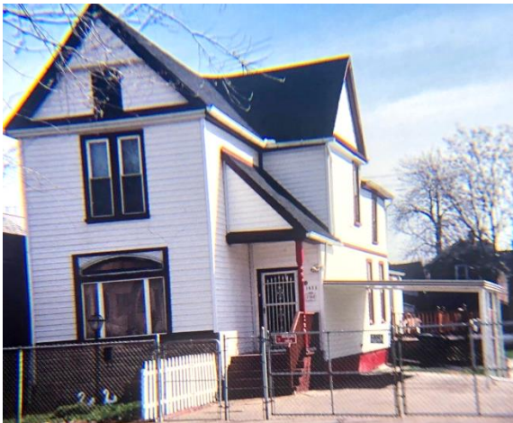
1984 Designation photo, HDAB.
