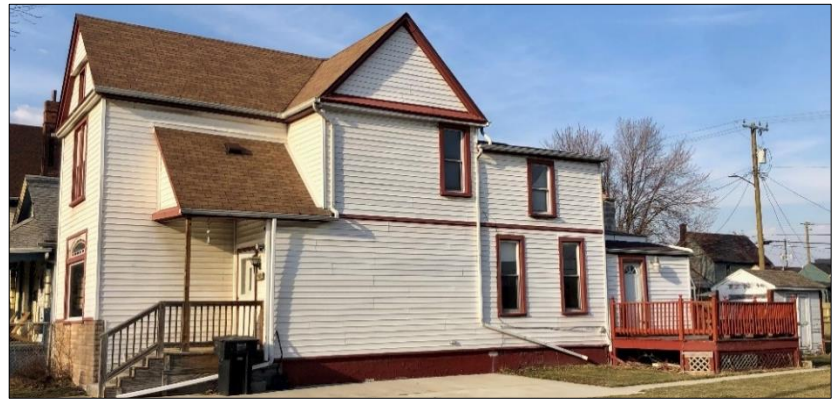
Top: Google aerial view, above: side (south) wall looking from Wabash.
