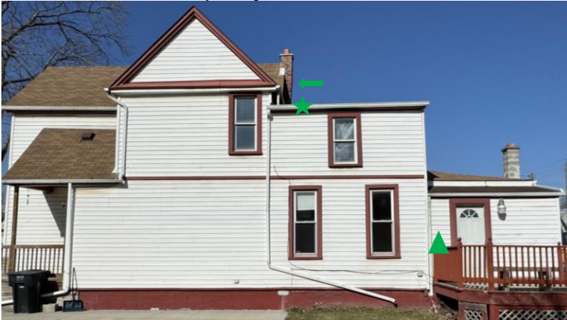
Existing south wall.
