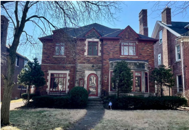
Site Photo 1, by Staff February 23, 2024: (North) front elevation.
