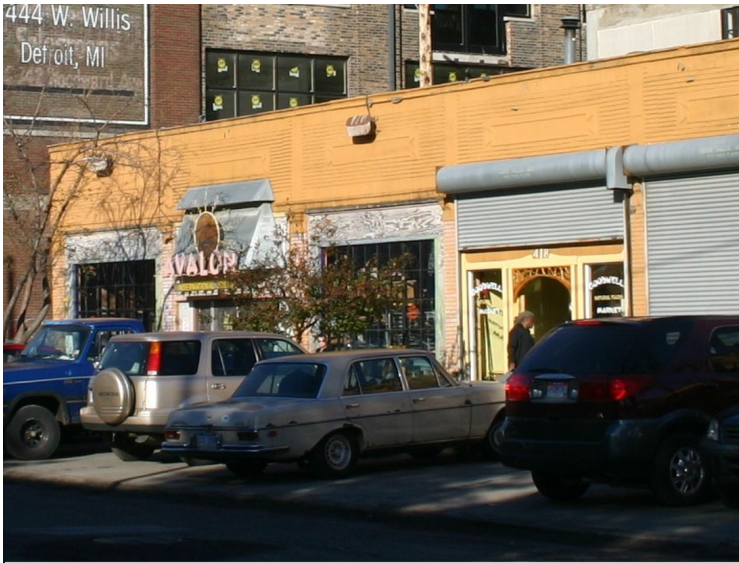
Site Photo 2, by Historic District Advisory Board, 2011: (North) showing painted masonry conditions at time of designation.
