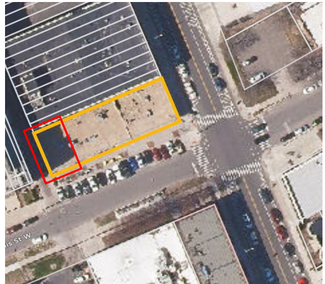
Aerial 1 of Parcel # 02002216 (in gold) by Detroit Parcel Viewer, the applicant has use of the space at 422 W WILLIS, shown in red.
