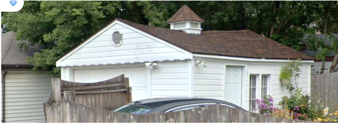
15301 Stahelin 1952/10/10 Garage ($644) // Dwelling – 1952/03/31 – 7 months between permits
