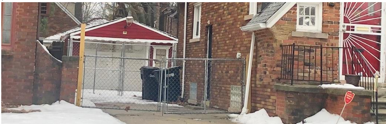
14907 Penrod – 1963 Garage ($896) // Dwelling – 1928/05/22 – 1950 Sanborn showed a garage in place but was not included on 1928 dwelling permit. Therefore, previous garage was likely erected at a different time than the dwelling, and the existing garage replaced earlier structure.
