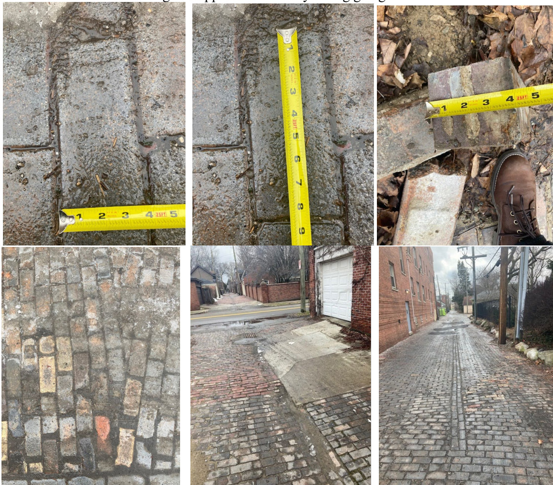
Figure 5: Images showing the dimensions and conditions of the paving in the alleys south of Lafayette.
