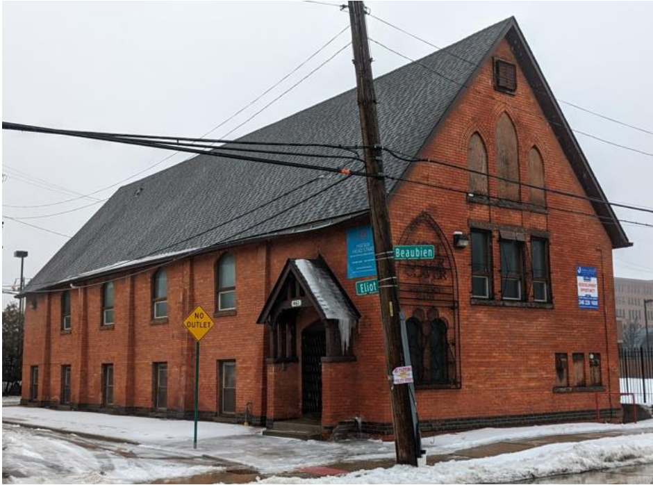
461 Eliot, viewed from southeast. January 2024 photo by staff.
