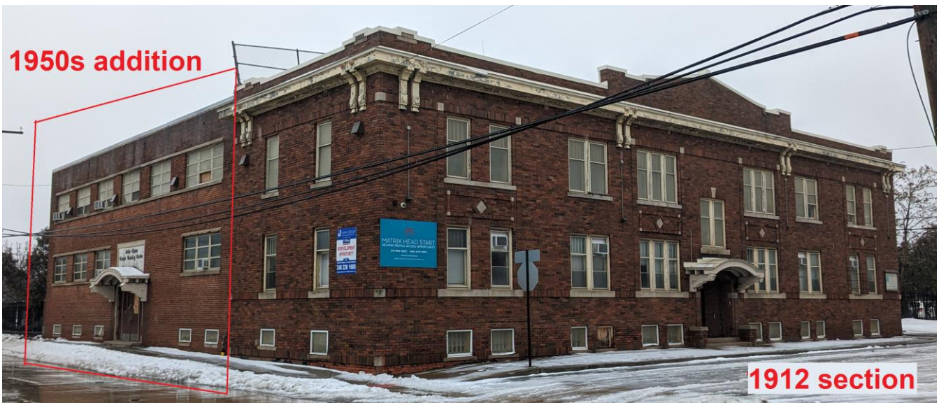
450 Eliot, viewed from northeast. The original 1912 section, depicted on the Sanborn map (page 3) occupies the foreground of the photo and faces north onto Eliot. The addition continues south along Beaubien. January 2024 photo by staff.
