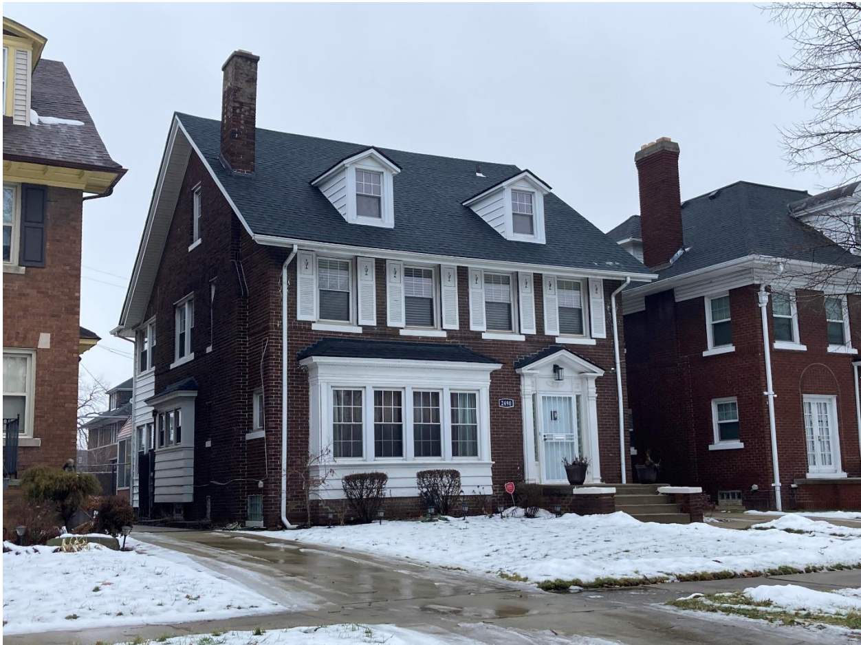
2490 Longfellow, note that the current windows are vinyl and aluminum coilstock is located at the window trim. 1/25/2024 staff photo
