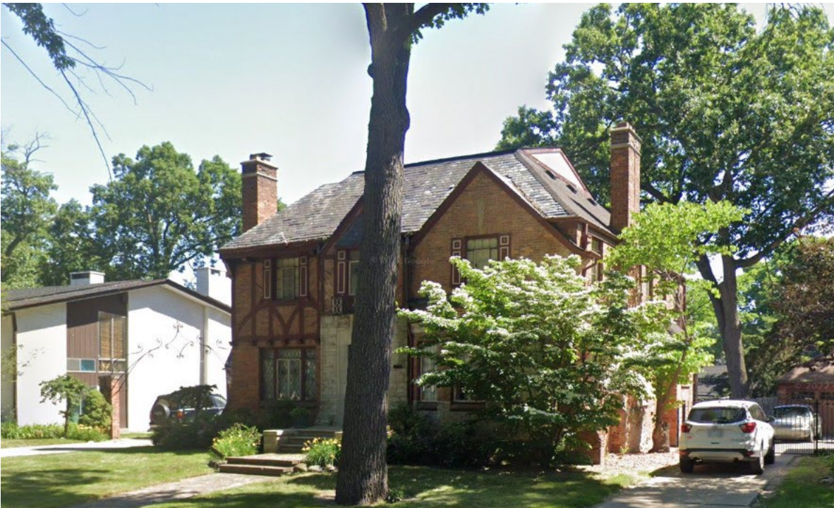
Figure 2: Image of 19650 Canterbury from 2019, showing the partial replacement of the slate roof at the side elevation. Google Street View
