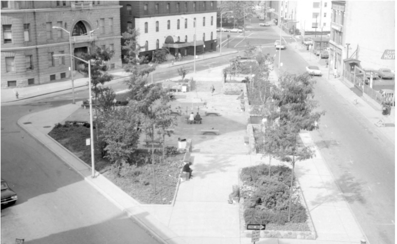
Site Photo 2 by WSU 1968, showing park conditions twenty years prior to historic designation in 1988, showing young honey locusts, low growing plantings within the planting beds and stone walls. Harmonie Club is located at the upper left.
