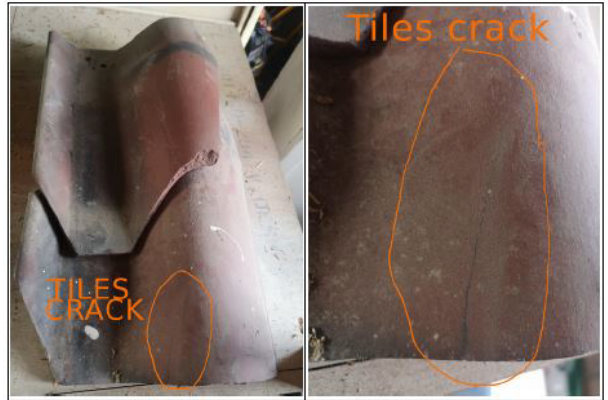
• 4) Description of Existing condition.
