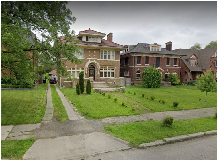
Site photo 2, by Google Street, June 2019: (Northwest) front showing original clay tile roof, driveway and sidewalk.
