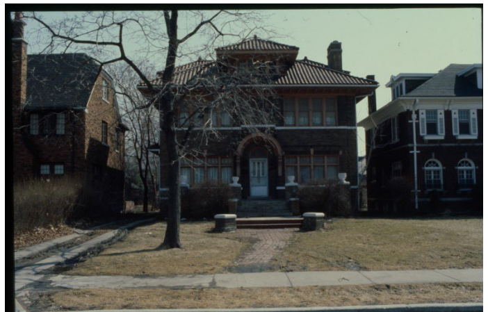
Designation Image, 1980: (Northwest) front elevation, showing original clay tile roof.
