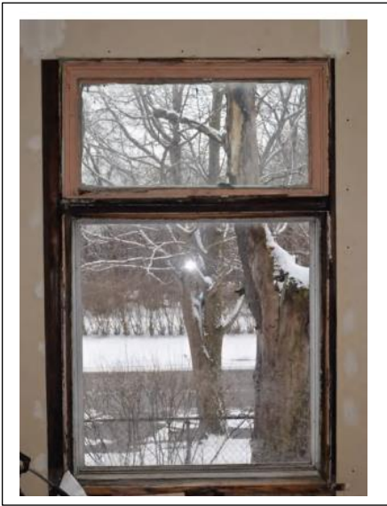
Fixed window with fixed transom at first story, 2021 condition (left) and 2023 condition after unapproved removal (right). The entire window and transom have been removed. The exterior woodwork remains
