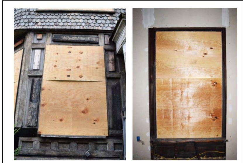
Fixed window with fixed transom at first story, 2021 condition (left) and 2023 condition after unapproved removal (right). The entire window and transom have been removed. The exterior woodwork remains
