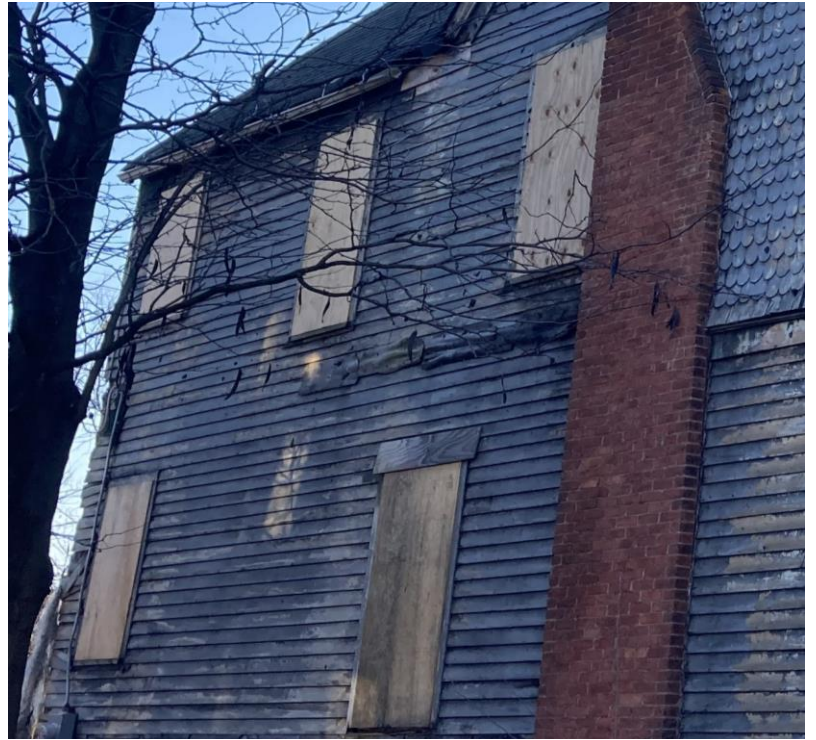
North wall. Appearance in 2021 (left) and 2023 (right). Note that these windows were single, 1/1 wood windows (with aluminum exterior storms). The 2021 application proposed to retain and restore these windows. The window sash at this wall has been removed while the exterior trim/casing remains.
