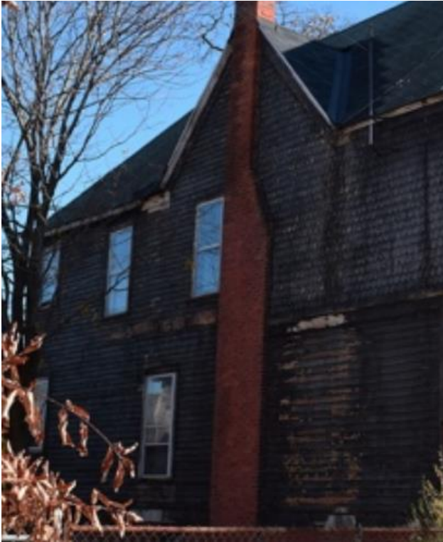
North wall. Appearance in 2021 (left) and 2023 (right). Note that these windows were single, 1/1 wood windows (with aluminum exterior storms). The 2021 application proposed to retain and restore these windows. The window sash at this wall has been removed while the exterior trim/casing remains.
