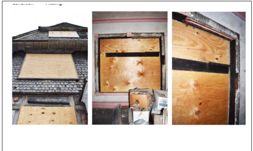
Paired mullioned double-hung windows with fixed transom at second story, 2021 condition (left) and 2023 condition after unapproved removal (right). The entire windows and to include horizontal and vertical mullions have been removed while the exterior casing and crown mould remains
