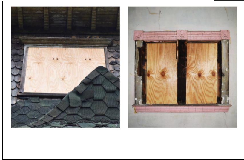
Fixed window with fixed transom at first story, 2021 condition (left) and 2023 condition after unapproved removal (right). The entire window and transom have been removed. The exterior woodwork remains
