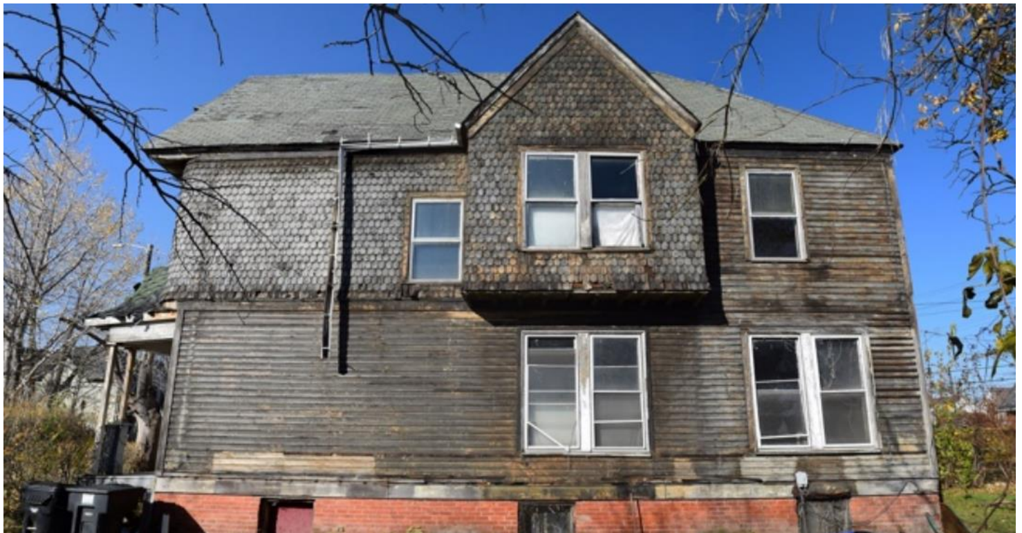
South wall, 2021. Note that this wall includes 1/1 wood windows (with aluminum exterior storm windows), both single and mullied, paired units. The 2021 application proposed to replace the window sash and exterior wood casing while retaining the mullions . The Commission approved this work item.
