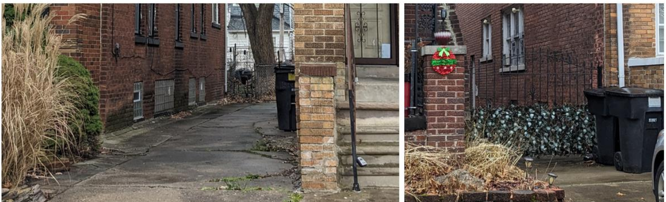
Left: Driveway spanned by a gate near the rear of the house and not readily visible. This configuration is common. Right: Driveway gate at the front plane of the house. This is much less common but is also appropriate. November 2023 staff photos.
