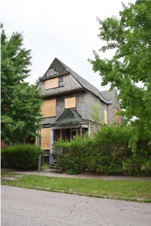
Front Façade looking North
