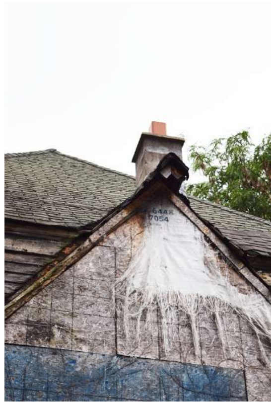
Rear coal chimney proposed for removal
