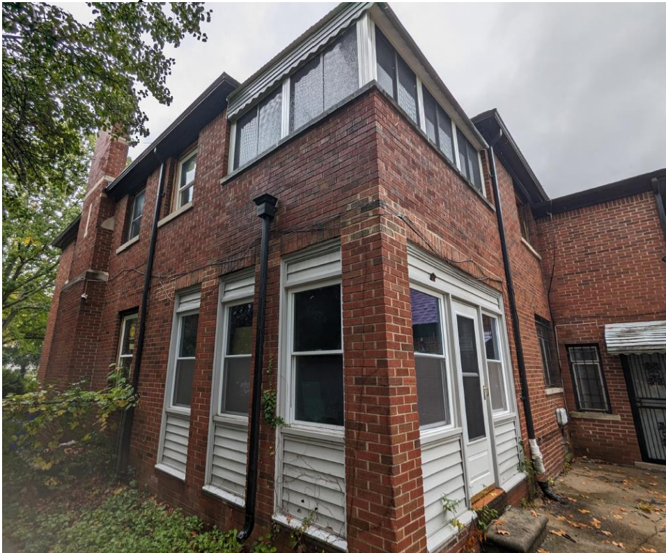
Applicant photo. Based on the masonry design of this rear corner, staff believes the upper area was possibly an open porch originally, and the lower area was possibly a screened enclosure. The vinyl window units within the first floor openings appear to be newer than the siding enclosure; the 2018 image on the preceding page shows vinyl units and the enclosed openings were in place at that time. Staff doesn't have earlier photo documentation of this area, but enclosures of porches in the 1950s-1980s were very common, so it is possible these enclosures pre-date district designation.
