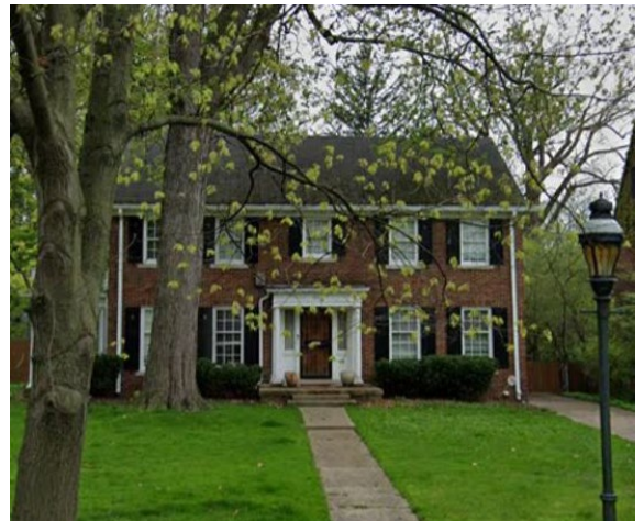
Site Photo 7, by Google Street May, 2019: 2211 Burns showing rectilinear modest porch steps and deck.
