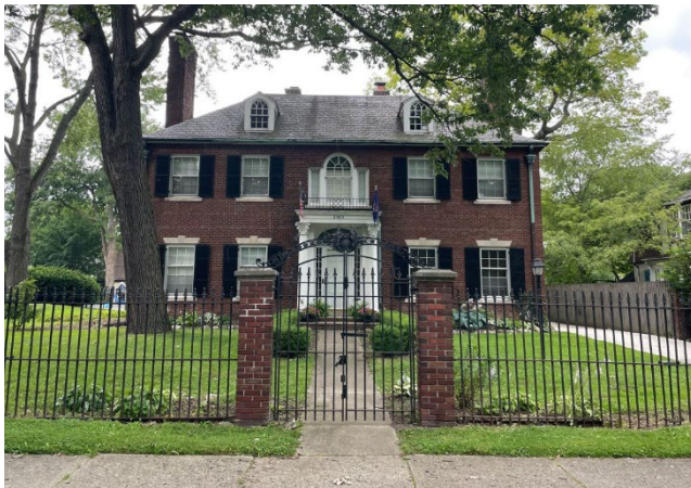
Site Photo 1, by Staff July 20, 2023: (East) front elevation, showing the existing front porch.
