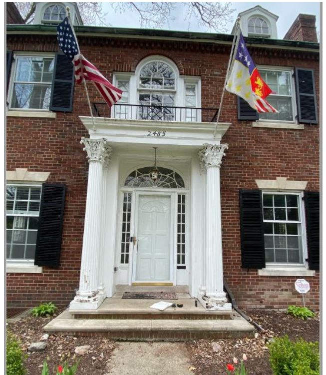
Site Photo 3, by Applicant: (East) front porch existing conditions, showing the original dimensions of the threshold, upper landing, and the lower step.
