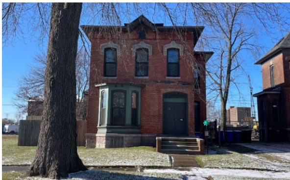
Site Photo 1, by Staff November 28, 2023: (East) front
