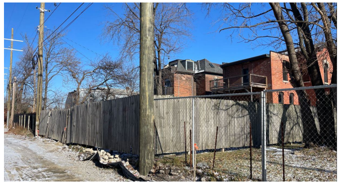
by Staff November 28, 2023: (west) rear elevation, showing existing fence to be removed and garage site along the alley.
