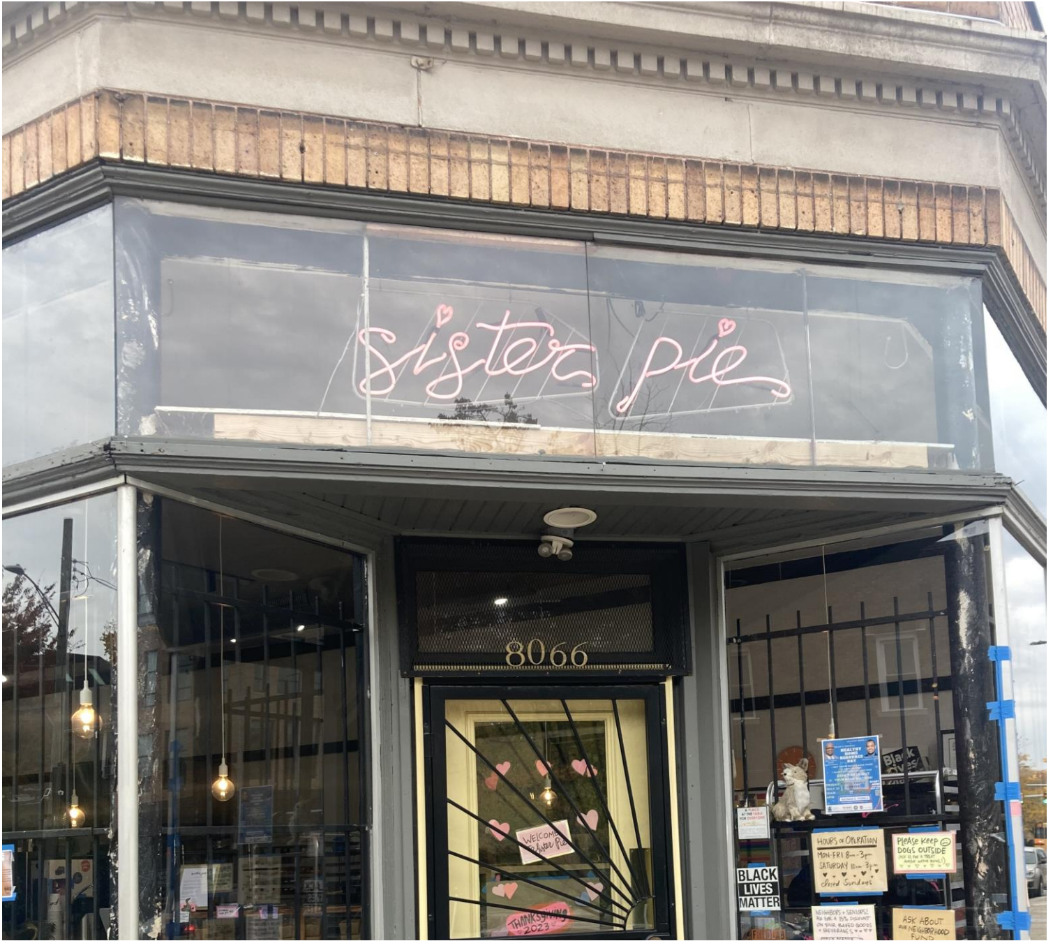
Transom at main entrance/primary storefront. Note trim profile. Staff photo taken 10/28/2023
