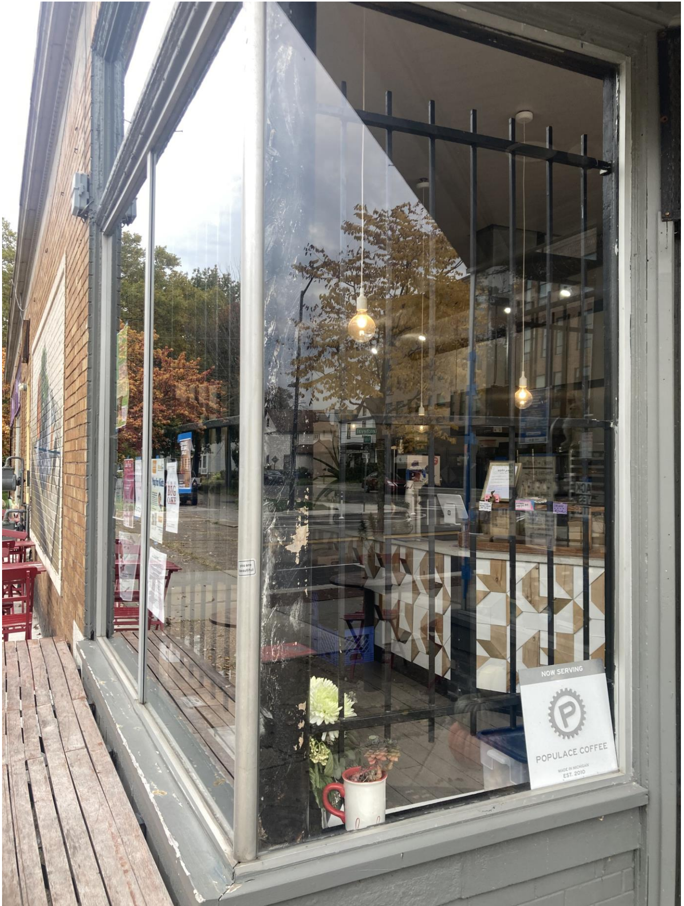
Storefront window at main entrance. The wood sill directly below the aluminum windows do not appear to be present in the 1983 designation slides. Staff photos taken on 10/28/2023
