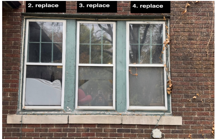
Site Photo 4, by Applicant, October 2023: (North) front elevation, first floor, showing original wood 6/1 windows behind storm windows for replacement.
