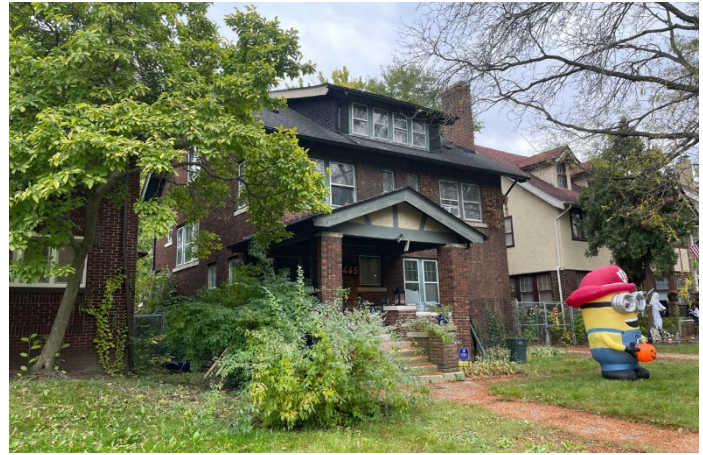
Site Photo2, by Staff, October 19, 2023: (East) side elevation of house, showing original wood windows behind storm windows.
