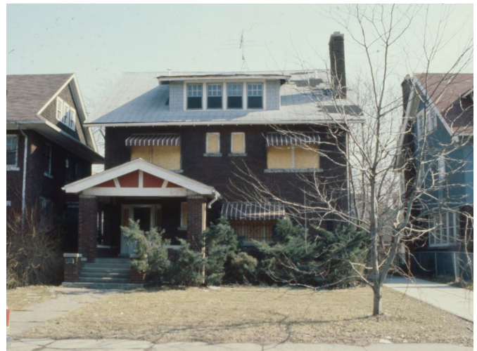
Designation photo 1980: (North) front elevation of the house showing 6/1 configuration in the dormer windows. Earlier designation photos are not available.
