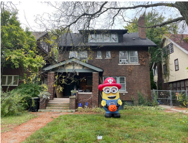
Site Photo 1, by Staff October 19, 2023: (North) front elevation of house, showing original wood windows behind storm windows.
