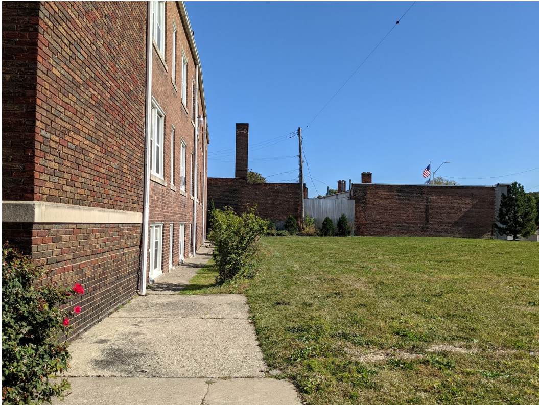
View to the east along south elevation of 1020 Alter, where loading drive is proposed. By staff's count, there are thirty-two (32) operable windows at this elevation, including several at grade. Staff Photo, October 1, 2021.
