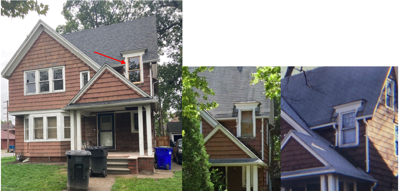
North Wall (Façade): One double-hung, wood sash window has been installed on the façade. This window was missing at the time the applicant purchased the home, but originally featured a leaded-glass upper sash with 12 lights.
