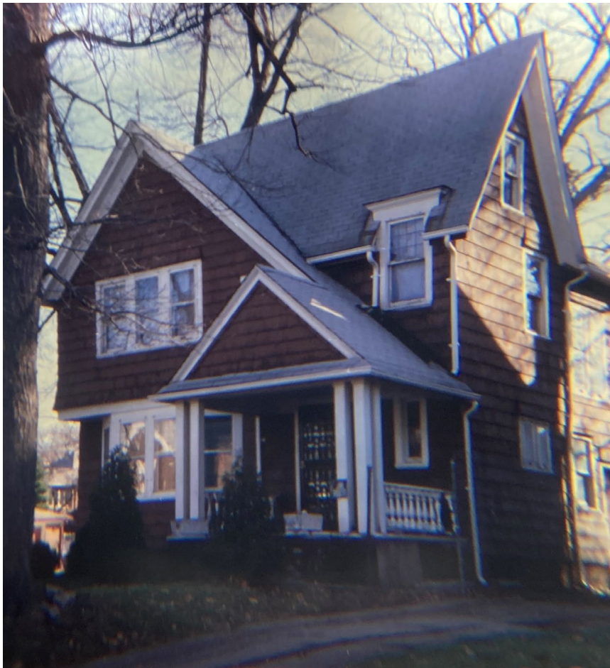
Figure 2: 4201 Glendale ca. 1999, looking southwest. HDAB
