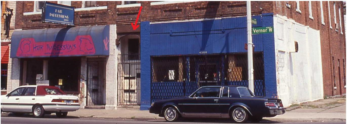
1993 Historic Designation Advisory Board photo, arrow added to indicate missing arch.
