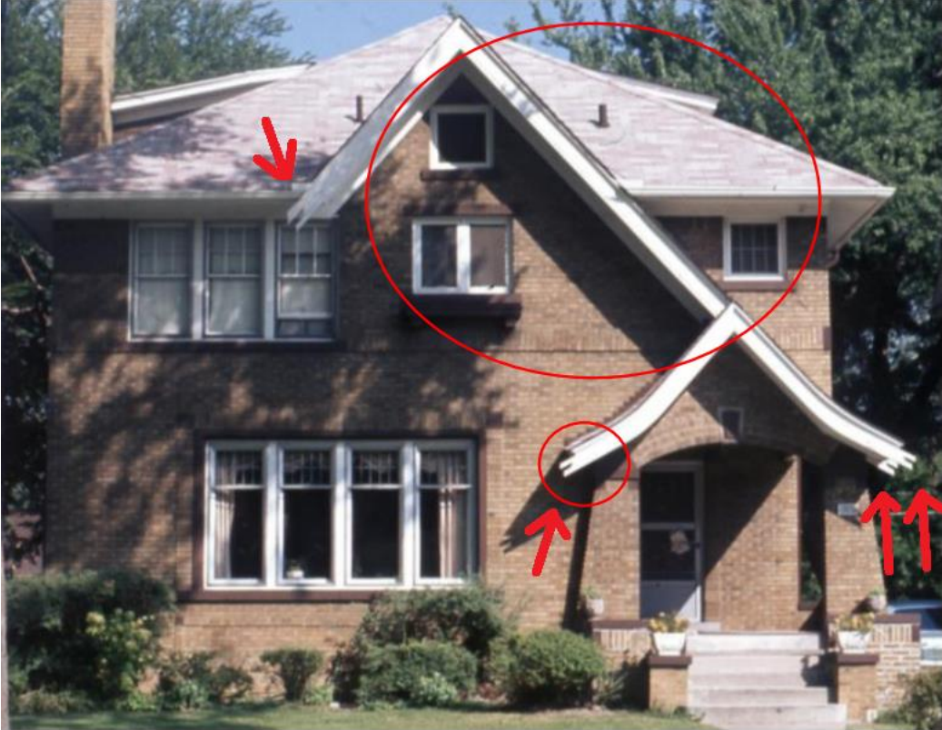
1974 photo by Historic Designation Advisory Board, notations added to highlight now-missing details.
