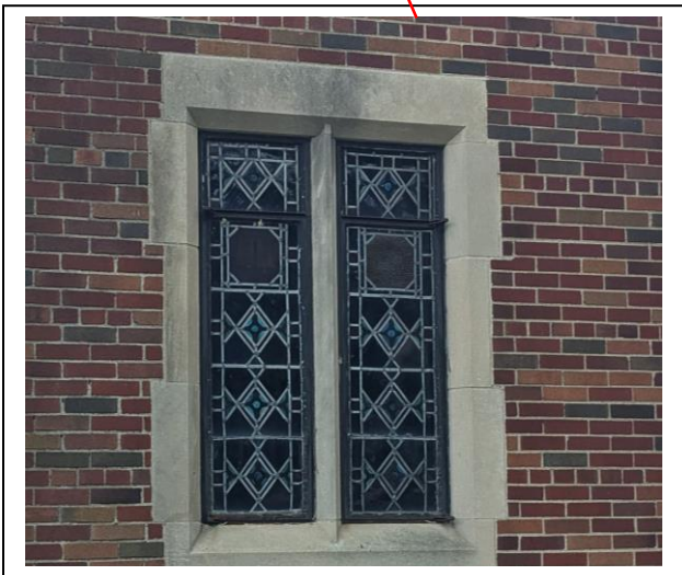
ORIGINAL STEEL CASEMENT AND TRANSOM WITH STAINED GLASS PANES (W/LEAD CAMING)
