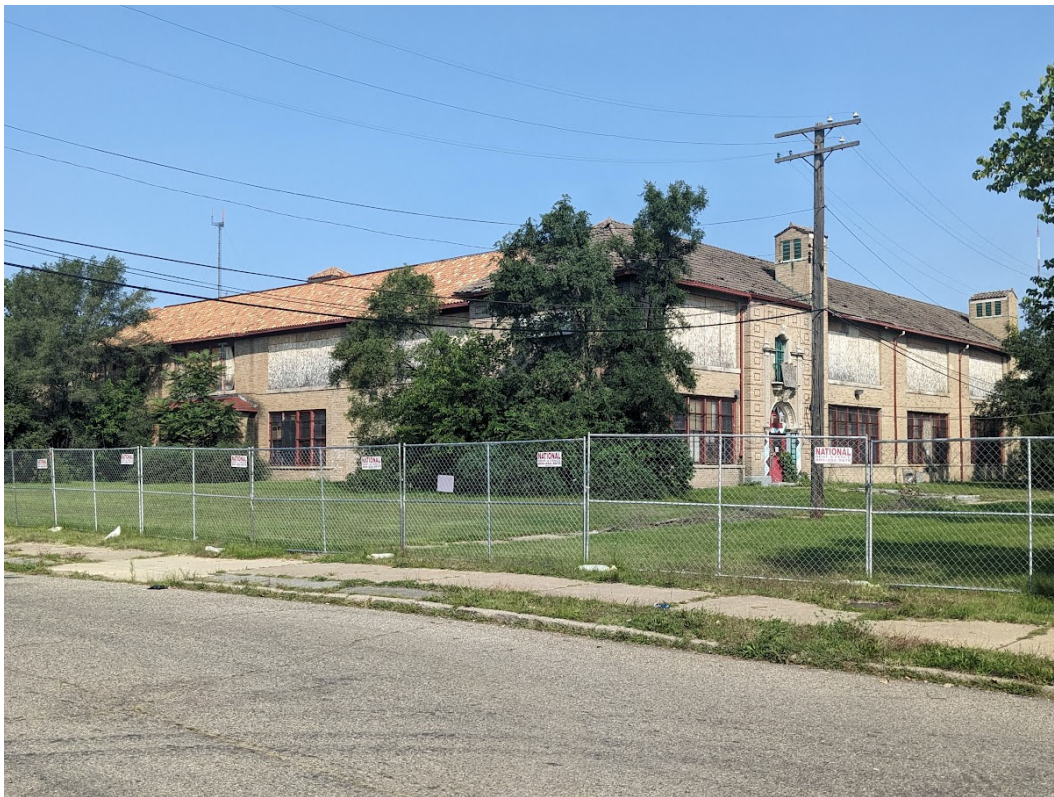
View of existing conditions at Higginbotham, looking to the northwest Staff photo, September 1, 2023.
