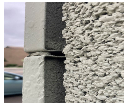
Site Photo 4, by Staff September 29, 2023 (front elevation): showing metal paneling detail.
