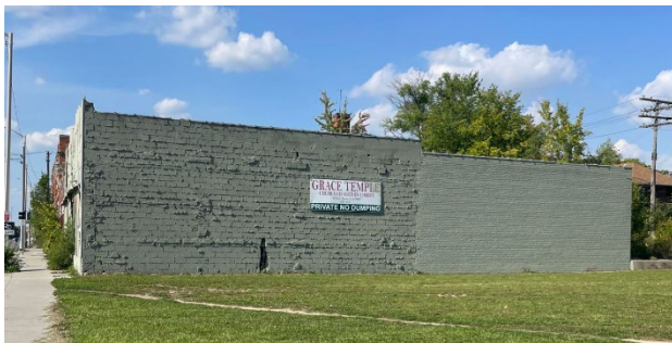
Site Photo 2, by Staff September 21, 2023: (South) side elevation, showing mural location.
