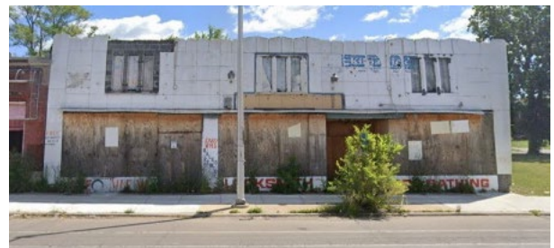
Site Photo 3, by Google Streetview June 2022: (West) front elevation, showing conditions prior to GSD painting the facade.
