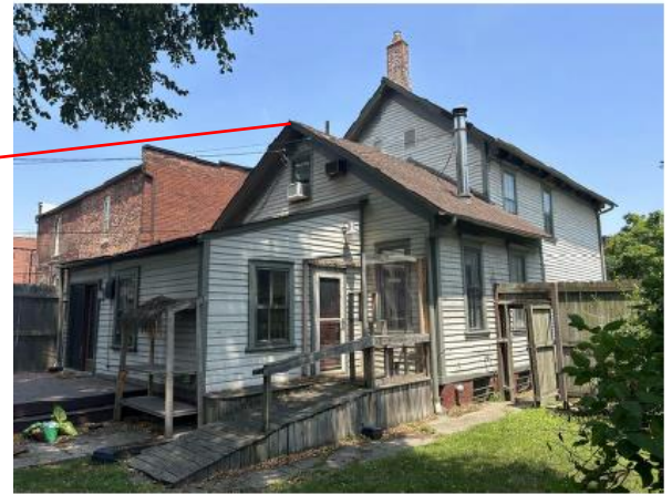
2. VIEW OF REAR LOOKING NORTHEAST (JULY 2023)
