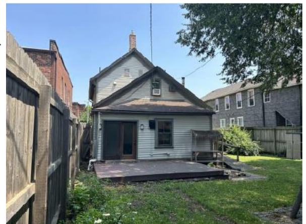
4. VIEW OF REAR LOOKING EAST (JULY 2023)
