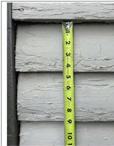
7. PHOTO OF EXISTING CONDITIONS
