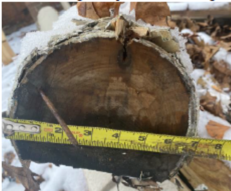
Diameter at the top of the pilaster – seven inches
