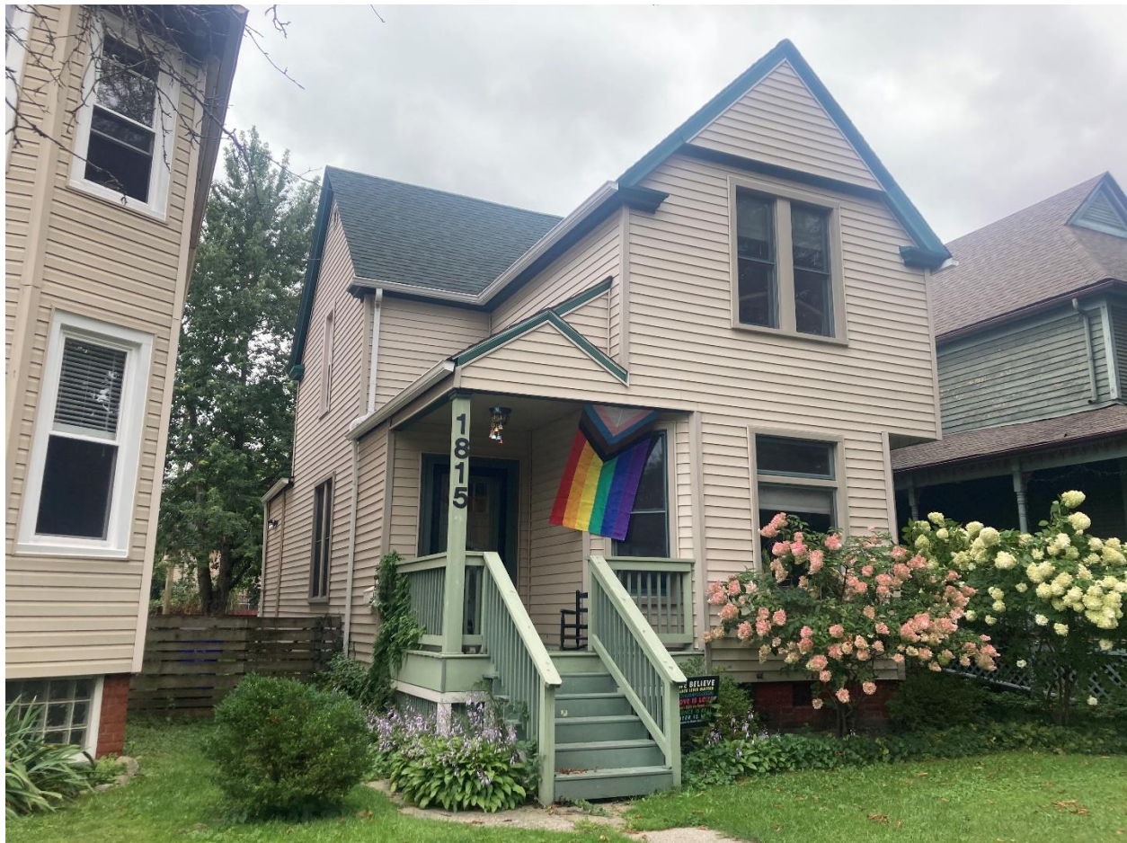
1815 Church, current appearance. Staff photo taken 8/31/2023
