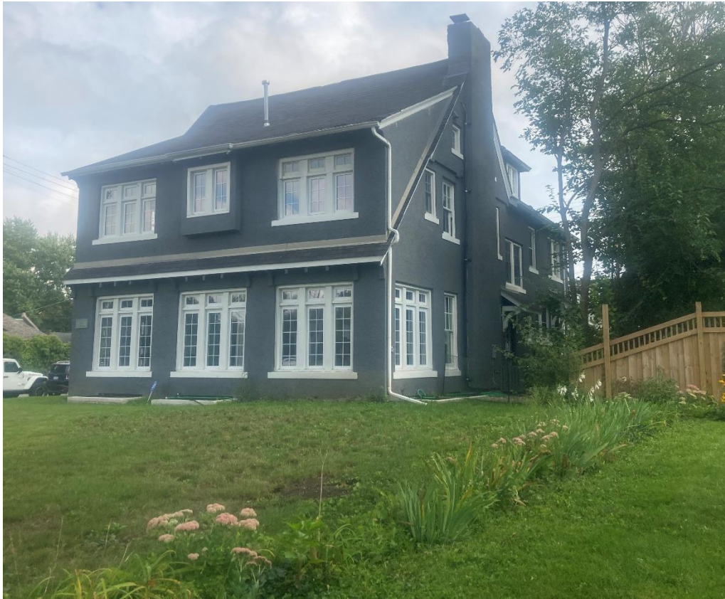
1405 Chicago Blvd., current appearance. Staff photos taken on 8/31/2023
