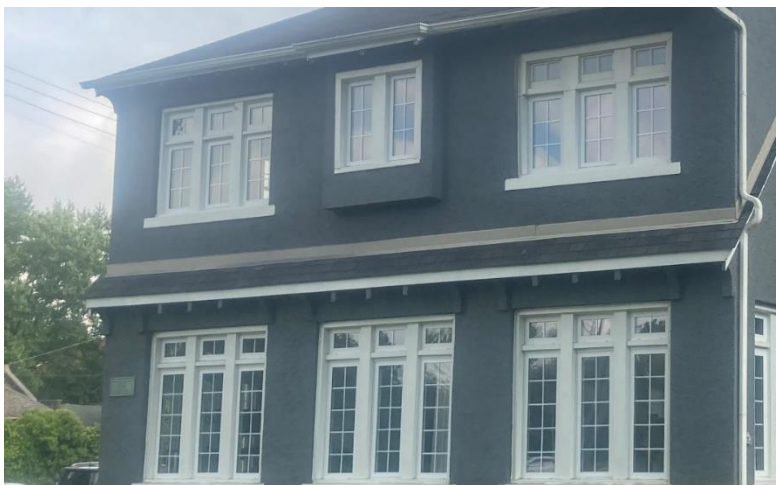
North side, current conditions
