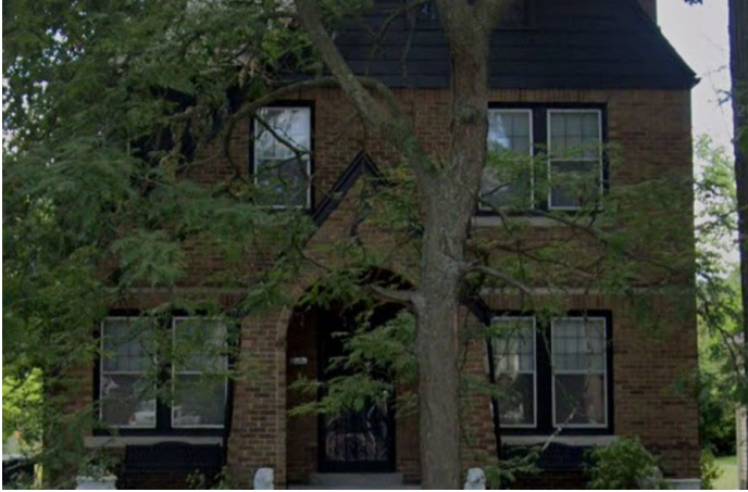
Site Photo 2, Google Streetview June 2022: (North) front/side elevation showing windows before work.
