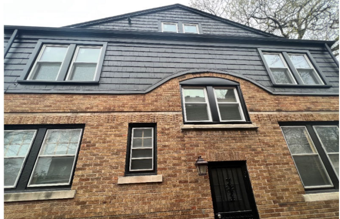
Site Photo 6, by Applicant, showing vinyl cover arch over vinyl window pair, located over the side entrance.
