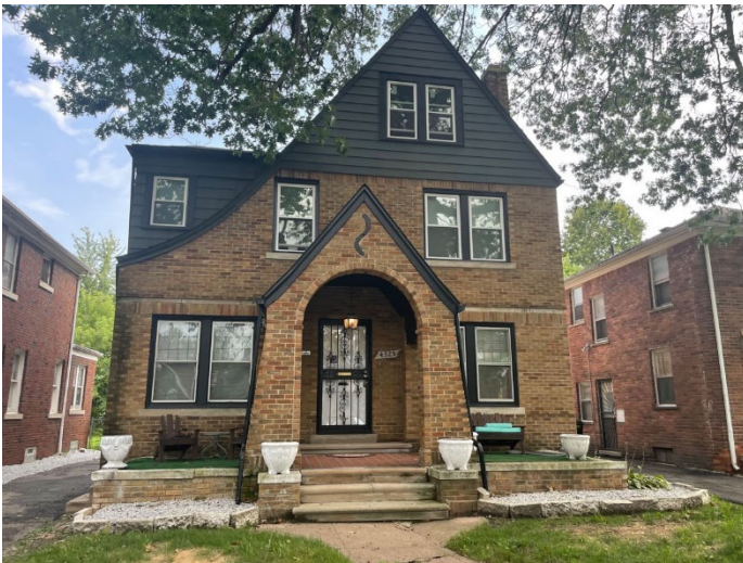
Site Photo 1, by Staff August 24, 2023: (North) front elevation showing replaced windows on 2 nd & 3 rd floors.
