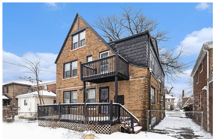
Site Photo 4, by Applicant 2022: (South) rear elevation showing replaced windows (unapproved) and approved repaired siding, new railings, and trim/siding paint work. Notice windows on 2 nd and 3 rd floor have been replaced, while the original first-floor windows remain.
