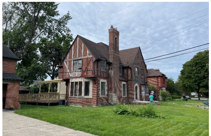
Site Photo 3, by Staff, August 14, 2023: East (side) and front elevation showing view of the deck, pergola and removed foundation plantings (without approval) from the public street.
