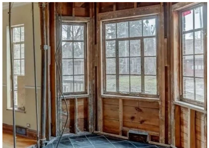
Site Photo 8, by realtor.com, April 2023: Dining room bay interior showing steel casement windows that were replaced by the current owner.
