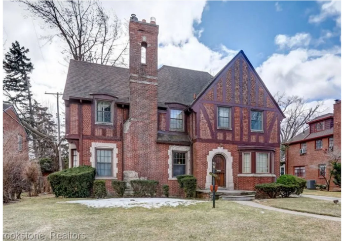
Site Photo 7, by realtor.com, April 2023: Front elevation (north) showing foundation plantings that screened the deck in the rear and casement windows at the east bay that were replaced by the owner.
