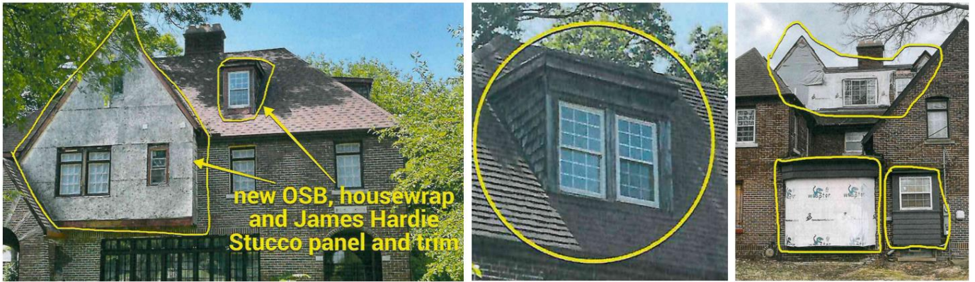
Proposed HardiePanel locations. Left to right: North elevation, west elevation, south elevation. Images by applicant.
