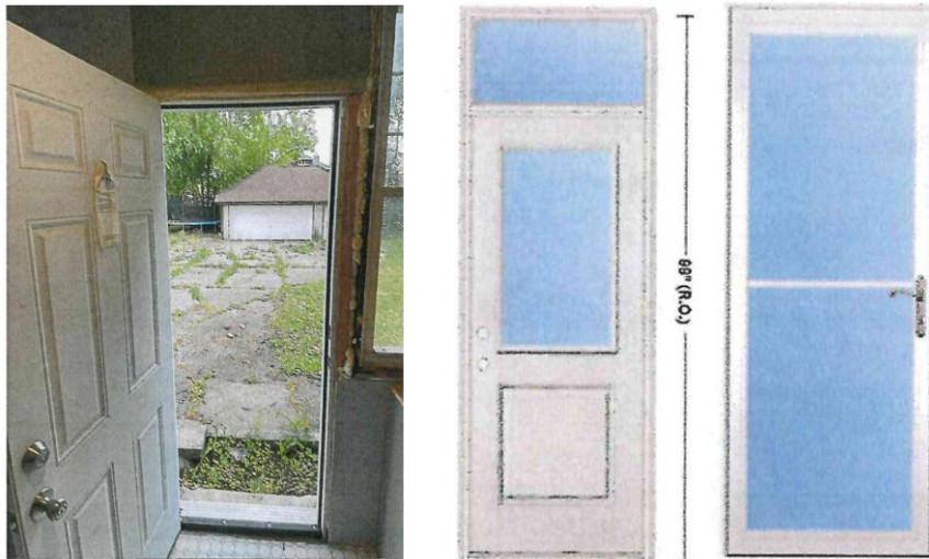
Left: Existing door. Photo from applicant. Center and right: Proposed door and storm door. Images from application materials.
