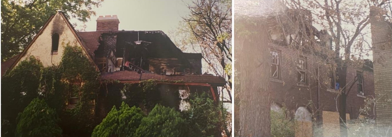
Left: North elevation in 2003. Right: West elevation in 2003. Staff photos from Historic District Commission files.
