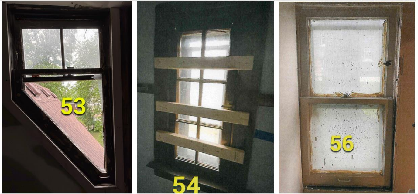
Examples of historic windows proposed for replacement.
