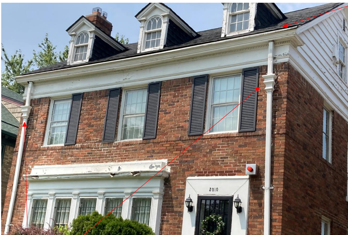
Current appearance. Staff photo taken on 7/18 /2023
