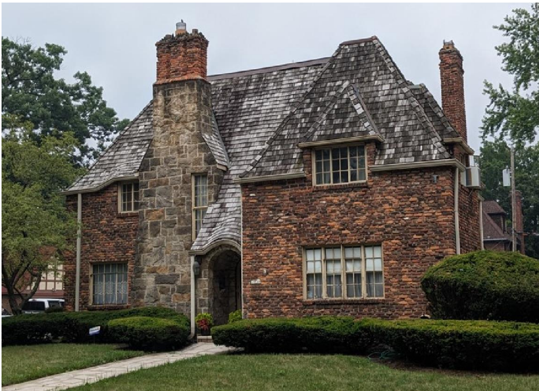
Front (southwest facing) view of subject property, June 2022 photo by staff.
