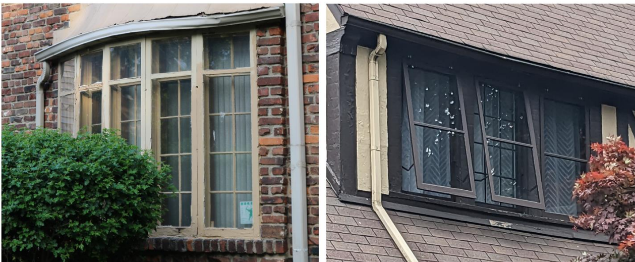
Left: storm windows on subject property. Right: storm windows on adjacent property. Photos by staff.
