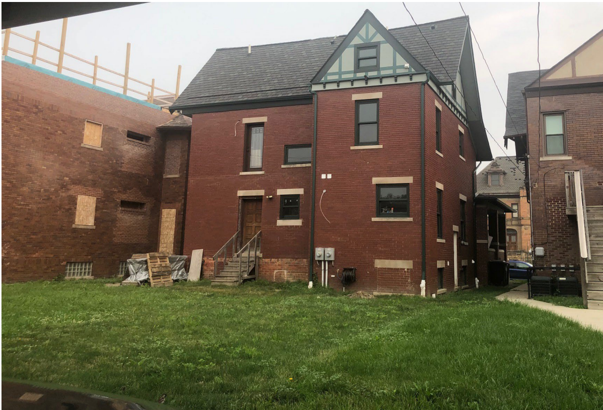
Staff photo, June 29, 2023. This zoomed-in view of 308 Eliot's rear elevation and yard was taken from the alley at the southwest corner of 314 Eliot.
