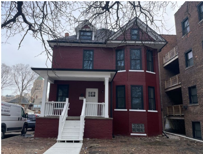
Site Photo 1, by Staff March 24, 2023: (North) front elevation.
