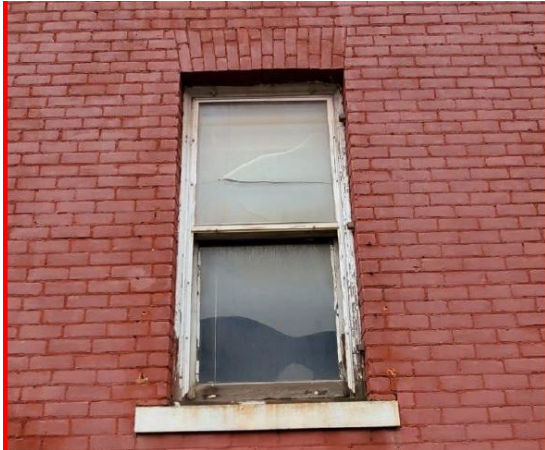
Site Photo 3, by Applicant 2019: (East) side elevation, showing original wood, double-hung window and depth of inset of the sash into the window opening.
