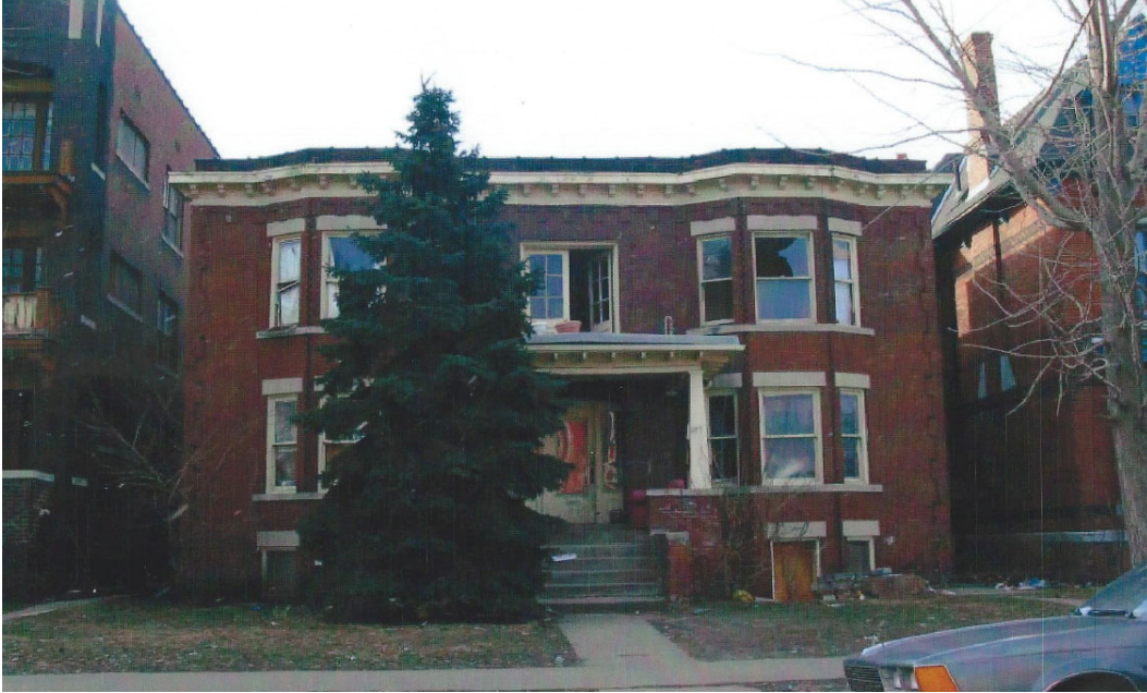
View of original historic building on the site, photo from 2004. Demolished 2018 as an emergency demolition.
