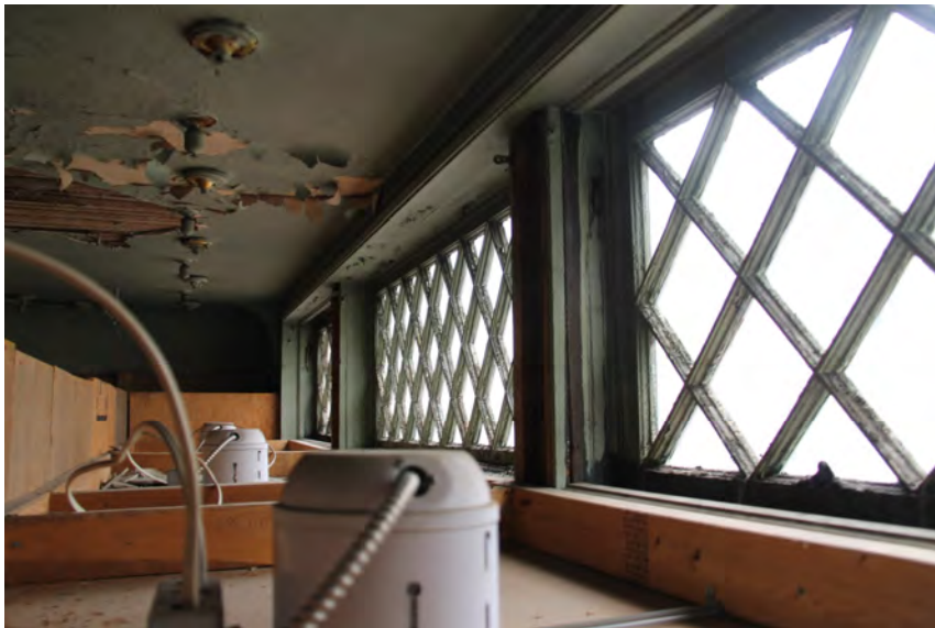
Interior 1336 Broadway, 2 nd Floor
