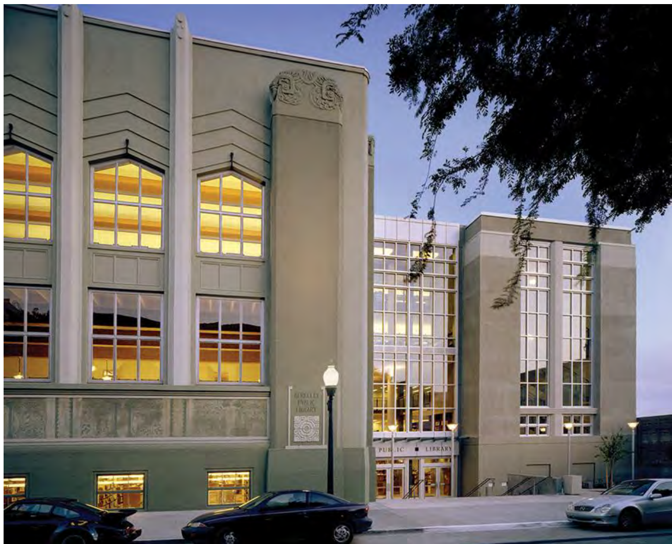
Figure 1. The addition to the right with its connecting hyphen is compatible with the Collegiate Gothic-style library. The addition is set back from the front of the library and uses the same materials and a simplified design that references, but does not copy, the historic building. Photo: David Wakely Photography.
