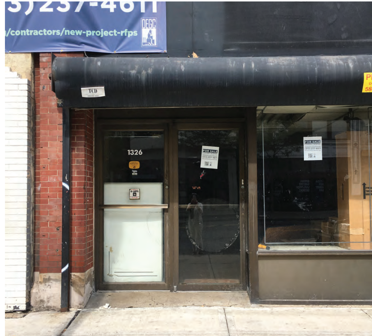
1326 BROADWAY SECURITY GRILL WILL BE REMOVED; NON-ORIGINAL STOREFRONT WILL BE RE- PLACED.
