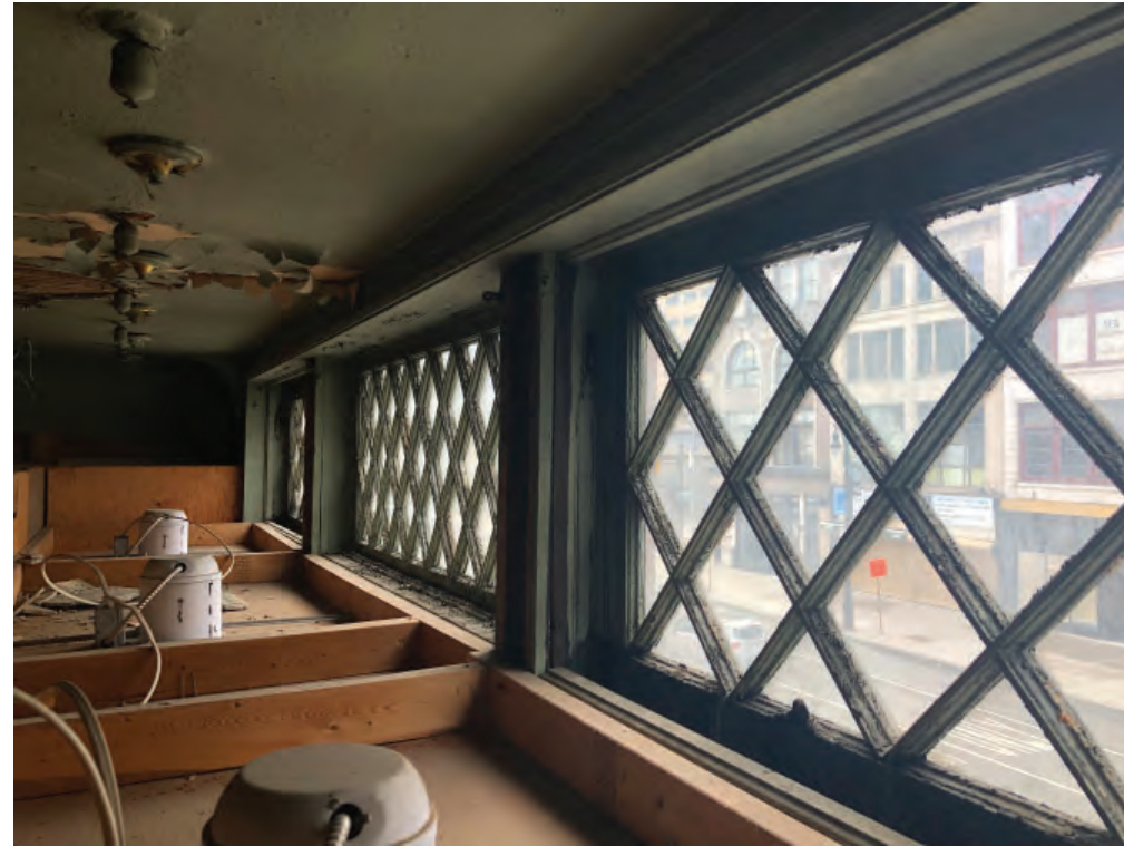
1326 BROADWAY 2ND STORY WOOD FIXED TRANSOM WINDOWS.
