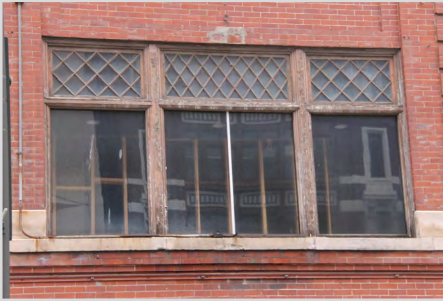
Window Front Façade 1336 Broadway, 2 nd Floor
