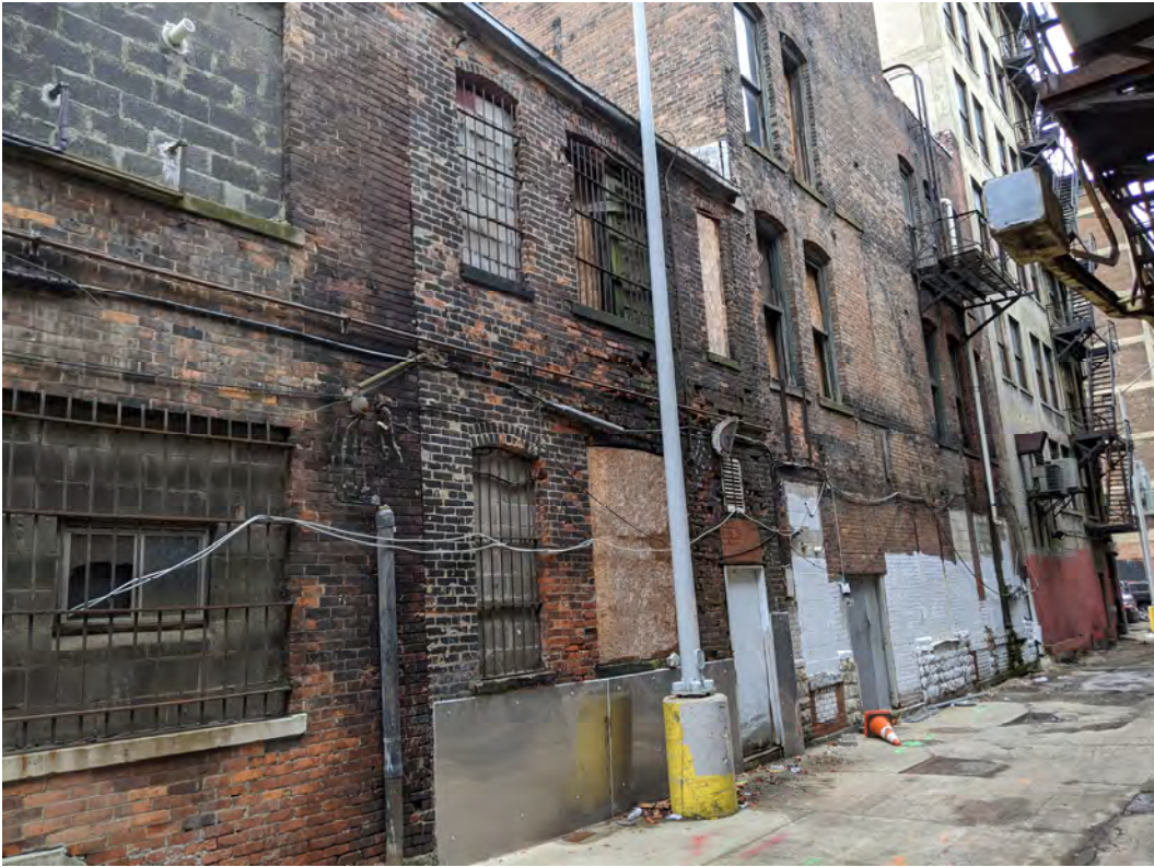
Rear of 1328-1332 Broadway, at alley. Staff photo, January 28, 2020.
