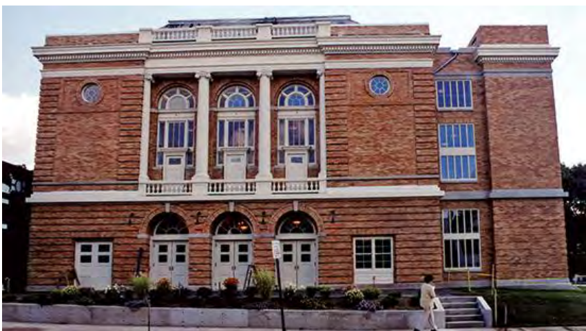
Figure 7. A vacant side lot was the only place a new stair tower could be built when this 1903 theater was rehabilitated as a performing arts center. Constructed with matching materials, the stair tower is set back with a recessed connector and, despite its prominent location, it is clearly subordinate and differentiated from the historic theater.
