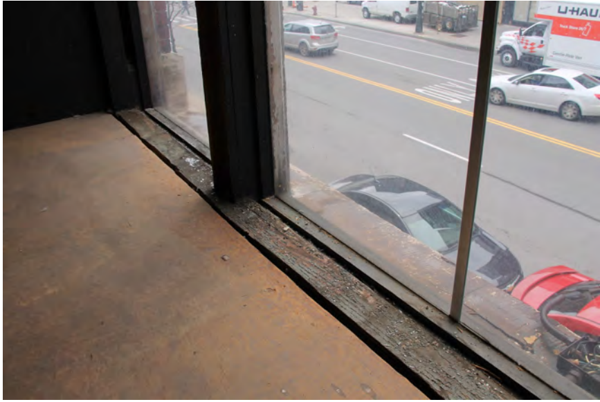
Interior 1336 Broadway, 2nd Floor
