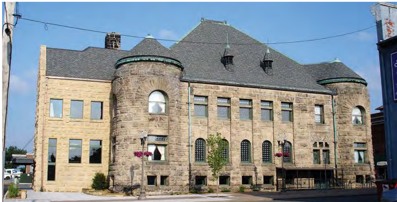
Figure 31. An elevator/stair tower was added at the back of this Richardsonian Romanesque-style theater when it was rehabilitated. Rough-cut stone and simple cut-out openings ensure that the addition is compatible and subordinate to the historic building. Photo: Chuck Liddy, AIA.
