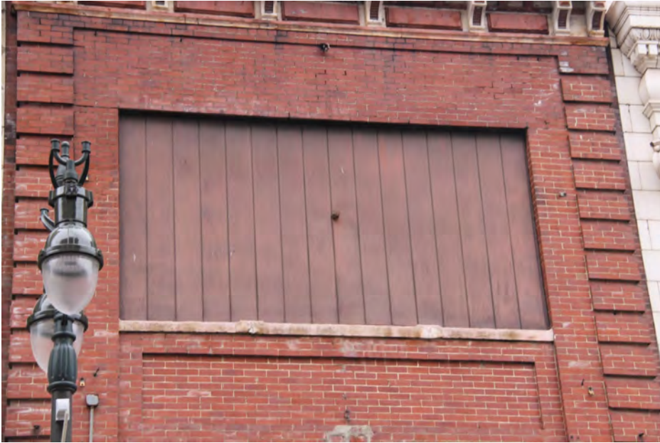
Window Front Façade 1336 Broadway, 3 rd Floor
