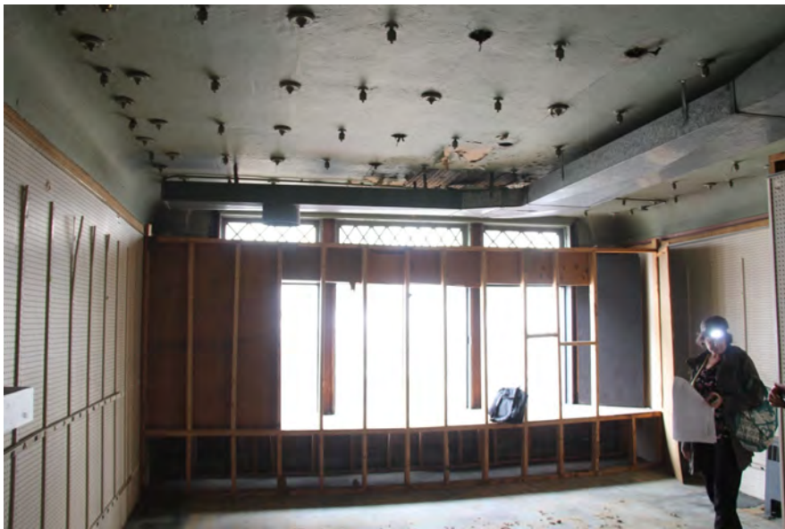
Interior 1336 Broadway, 2 nd Floor
