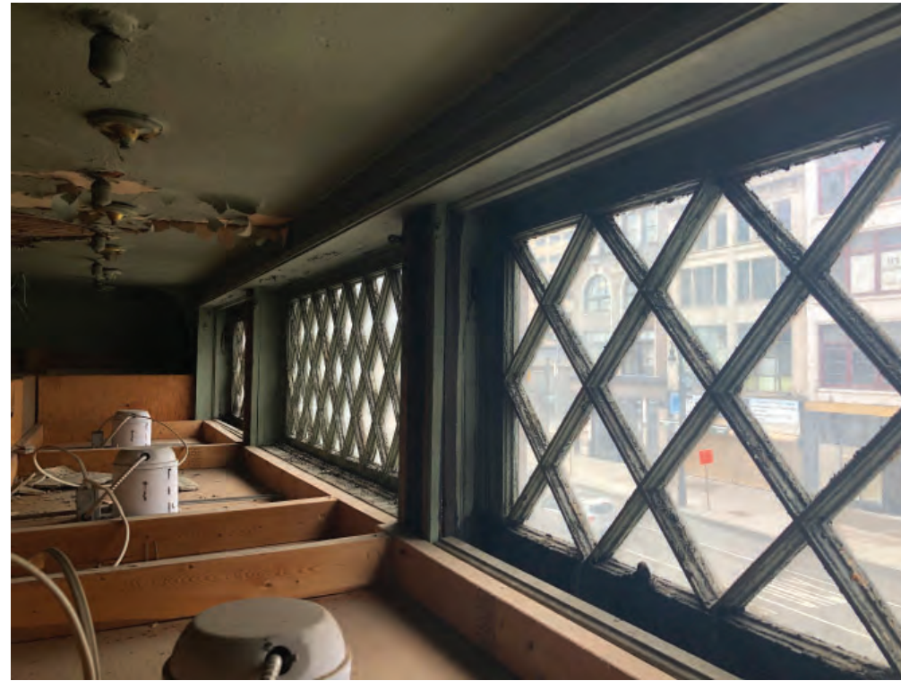
1326 BROADWAY 2ND STORY WOOD FIXED TRANSOM WINDOWS.
