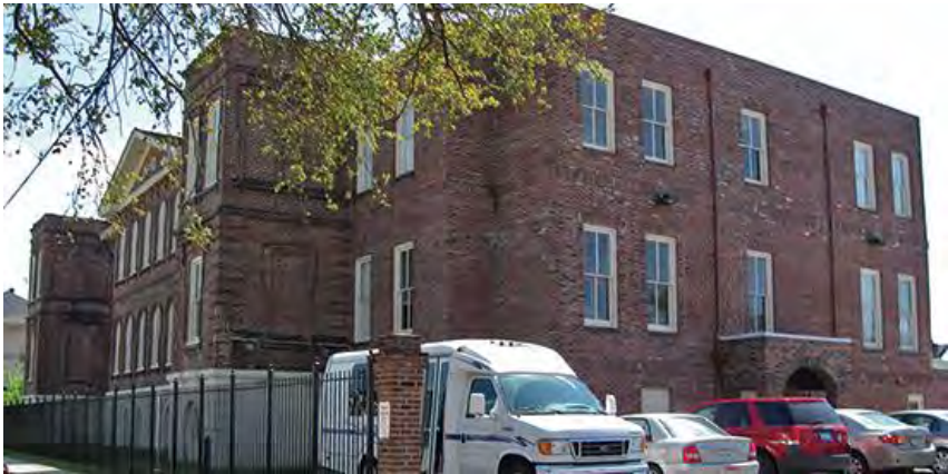
Figure 9. A simple, brick stair tower replaced two non-historic additions at the rear of this 1879 school building when it was rehabilitated as a women's and children's shelter. The addition is set back and it is not visible from the front of the school.
