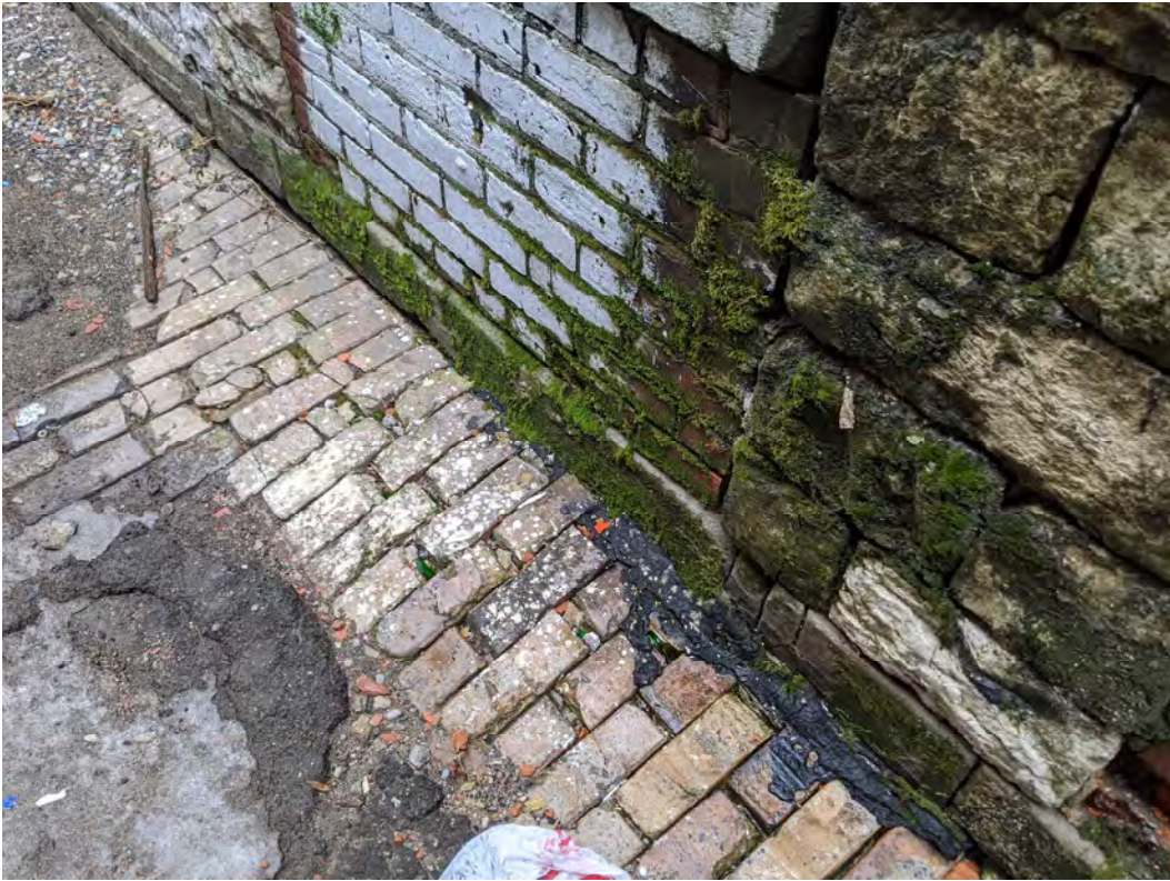
Detail view at rear of 1332, at alley. Staff photo, January 28, 2020.
