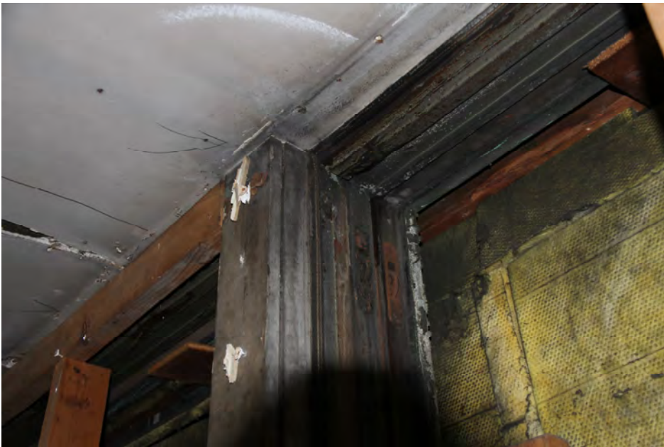
Interior 1336 Broadway, 3 rd Floor
