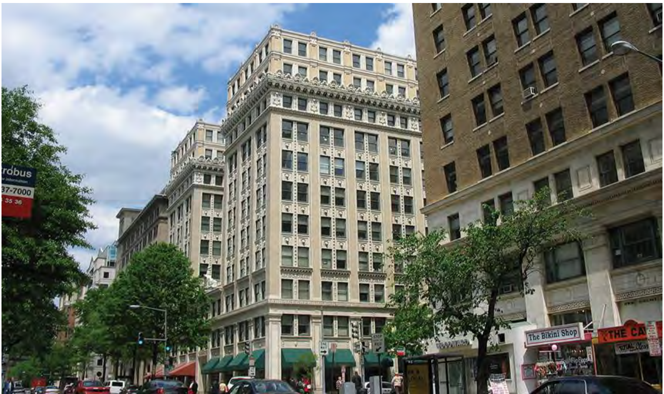
Figure 19. The upper two floors of this early-20th century office building were part of the original design, but were not built. During rehabilitation, the two stories were finally constructed. This treatment does not meet the Standards because the addition has given the building an appearance it never had historically.
