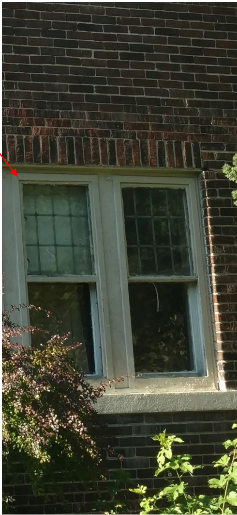
Figures 3,4: Photographs of the original windows (left), and extant replacement windows (right) on the side elevation of 535 Arden Park. The red arrow indicates the wood pieces the proposed project aims to replicate.
