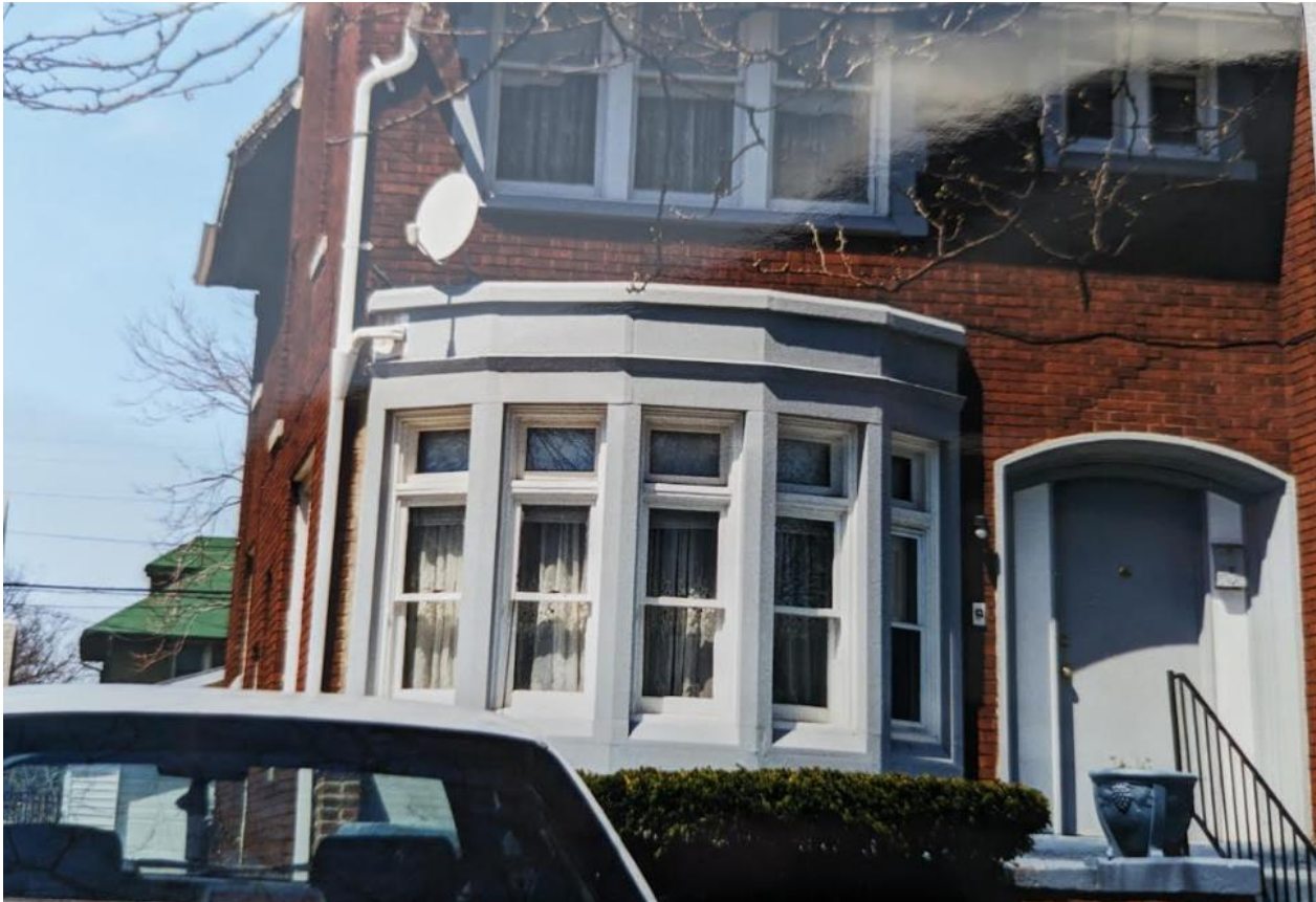
May 2000 staff photo. Note thickness and depth of window sashes differs from current windows. Note also the non-historic door.
