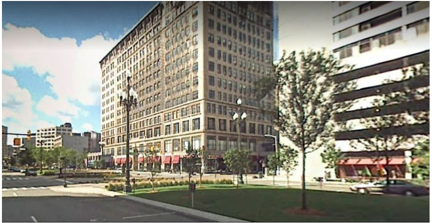
Figure 6, Washington Blvd. from Grand River Ave. looking south, ca.2007
