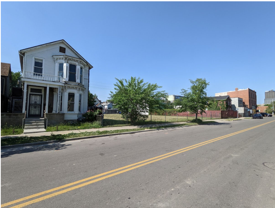
View of existing conditions at 1530 Bagley, looking towards the north. Development site is the vacant area at center. Staff photo, May 31, 2023.
