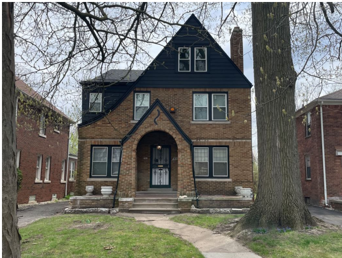
Site Photo 1, by Staff April 20, 2023: (North) front elevation showing replaced windows on 2 nd & 3 rd floors, black painted siding/trim, and removed light post.
