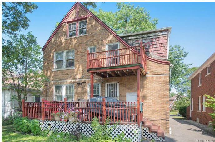
Site Photo 3, by Applicant (unknown date) March 22, 2023: (South) rear elevation, showing original windows, deck and balcony railing, siding, and trim colors.
