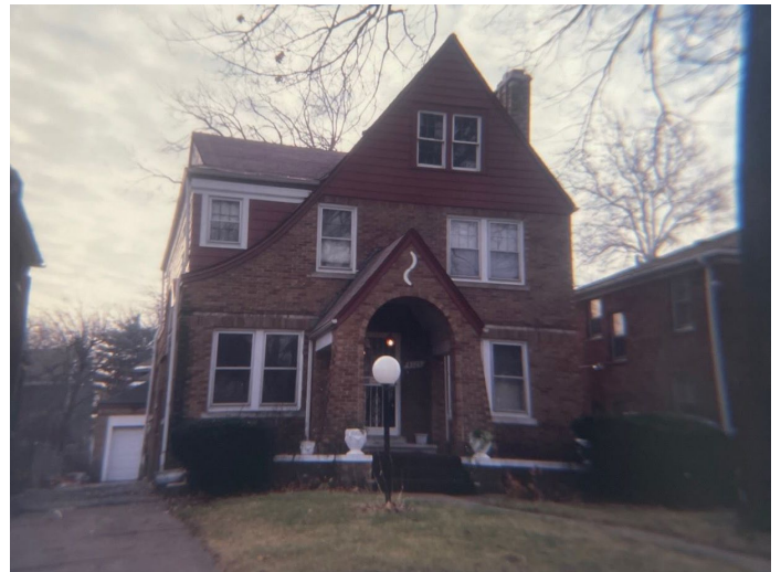
Designation Slide, 1999: (North) front/side elevation showing original windows and light post.
