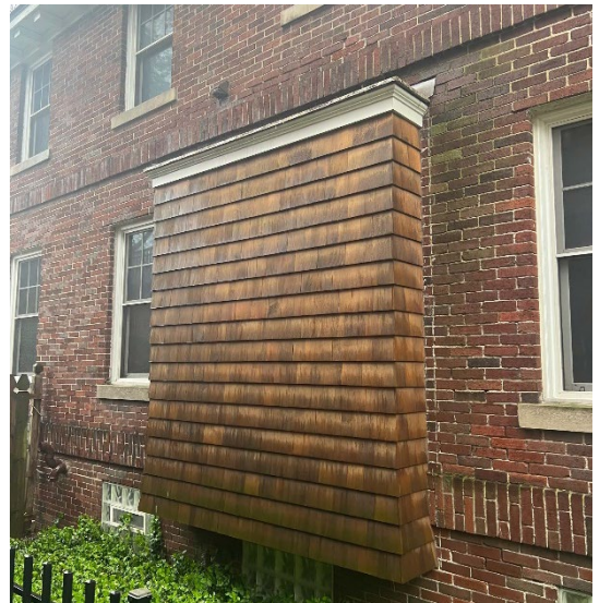
Site photo 5, by Applicant: (East) side elevation, showing cedar shake siding installation at bump-out.
