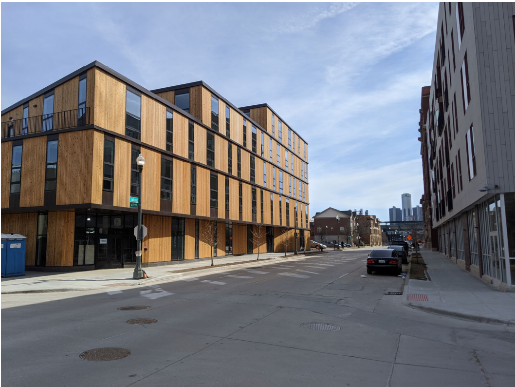
View along John R to south, showing recently constructed apartment building in vicinity. Staff photo.
