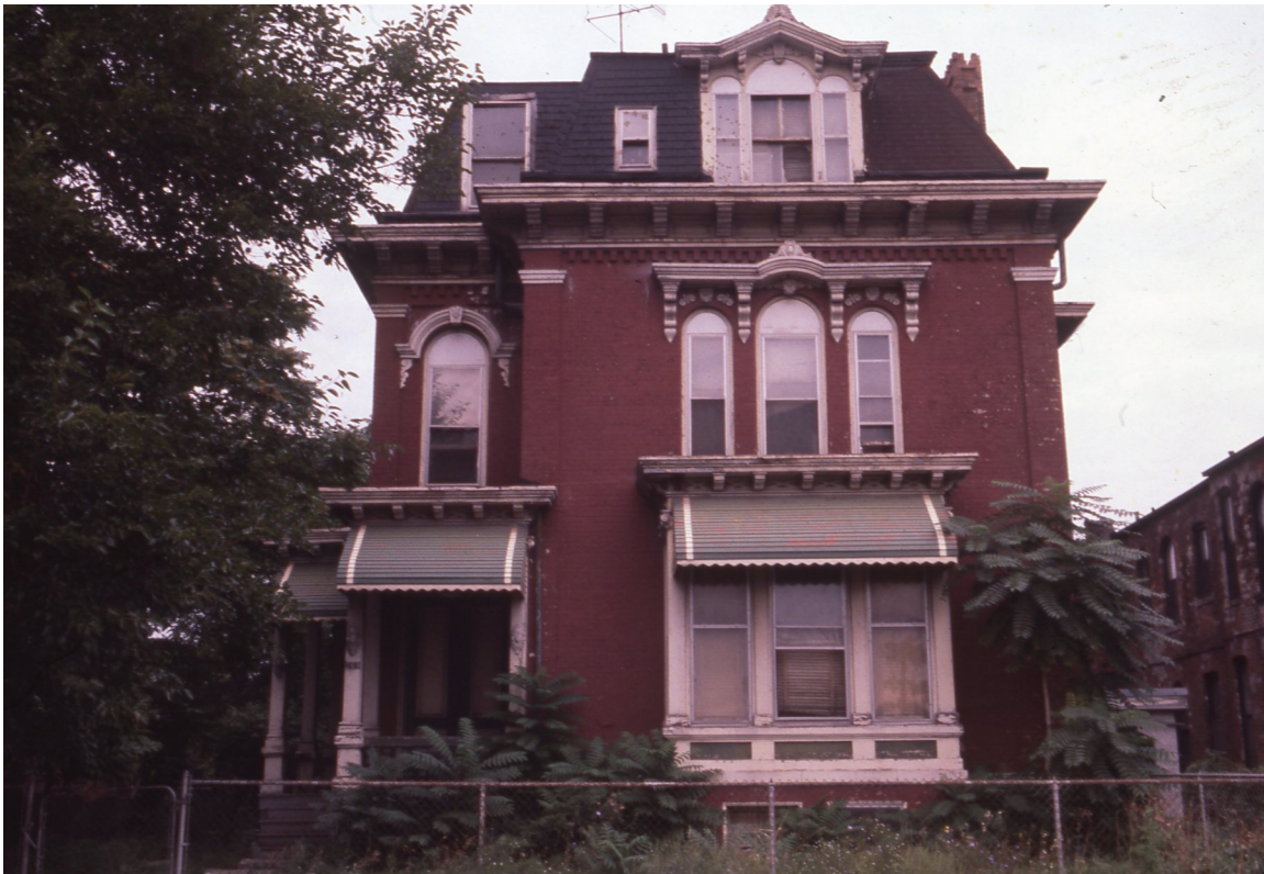
HDAB Designation Photo of 269 Winder, 1980. Demolished 2009.
