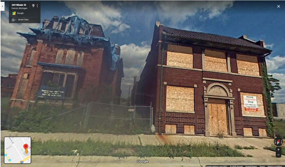
Google Street View photo of 269 and 281 Winder from 2007, about two years before demolition.
