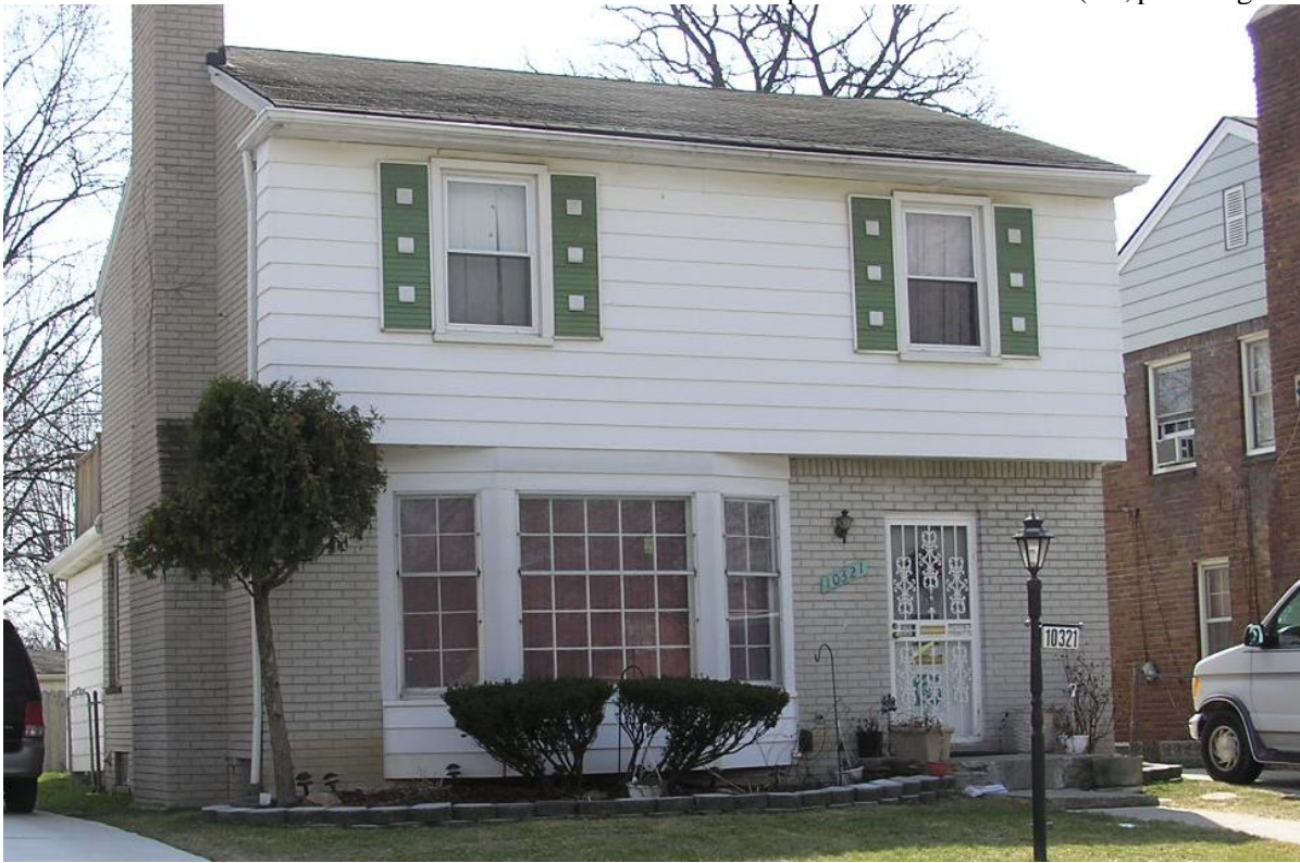
Designation photo, 2006, HDAB.
