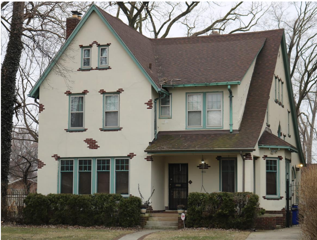
House at 3521 Seminole. March 2023 photo by staff.
